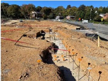
Concrete walls are being formed and poured for the fitness expansion area, under-slab utilities are being installed, and the concrete slab will be poured soon.
