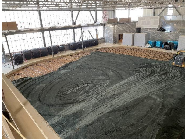
Left and Right: The new rink includes two layers of temperature-regulating lines. The lower lines (shown here) are frostshield tubing which, together with a 4" sand layer and a 3" insulation layer, will help maintain the temperature below the cooled concrete slab.
