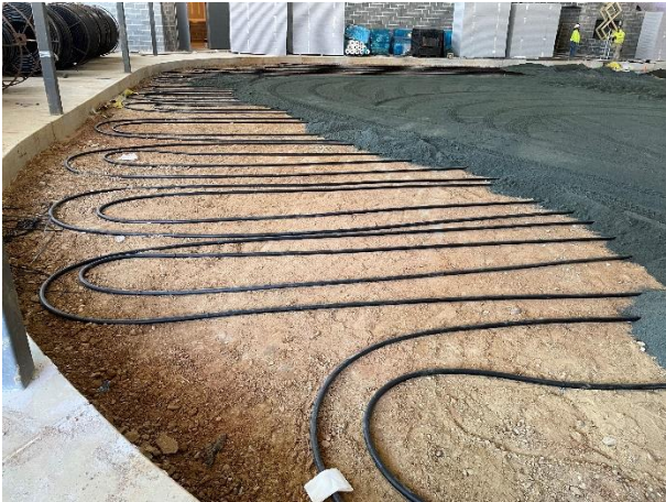
Left and Right: The new rink includes two layers of temperature-regulating lines. The lower lines (shown here) are frostshield tubing which, together with a 4" sand layer and a 3" insulation layer, will help maintain the temperature below the cooled concrete slab.
