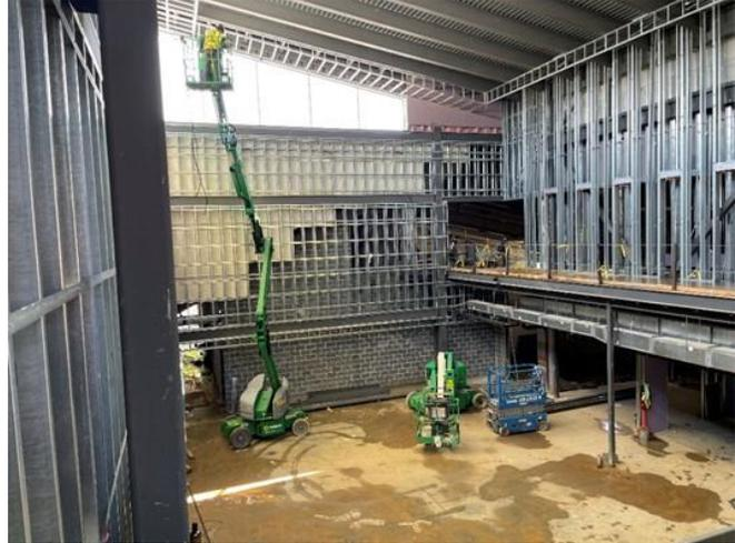
*Left:* Contractors are preparing the upper-level fitness area for siding and glass while masonry installation continues on the building and adjacent walls.
