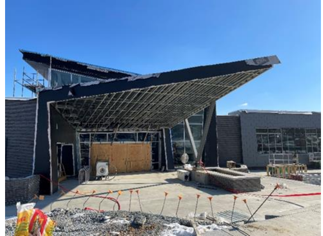
Left: The new NHL-size ice rink with metal panel installation in progress.
