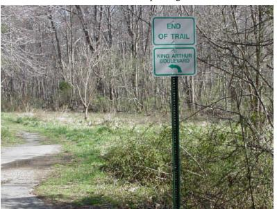
These signs are constructed of aluminum and marked with green letters or symbols on a white background. They may be mounted on u-channel posts, wood posts, or attached to fences, etc. A typical direction sign, constructed of 2" u-channel post with a 12"x18" aluminum sign is shown here.
