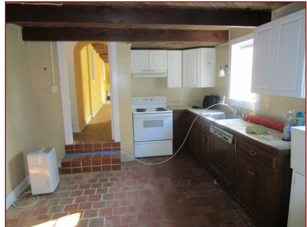
Image 8: Kitchen Condensate Piping
