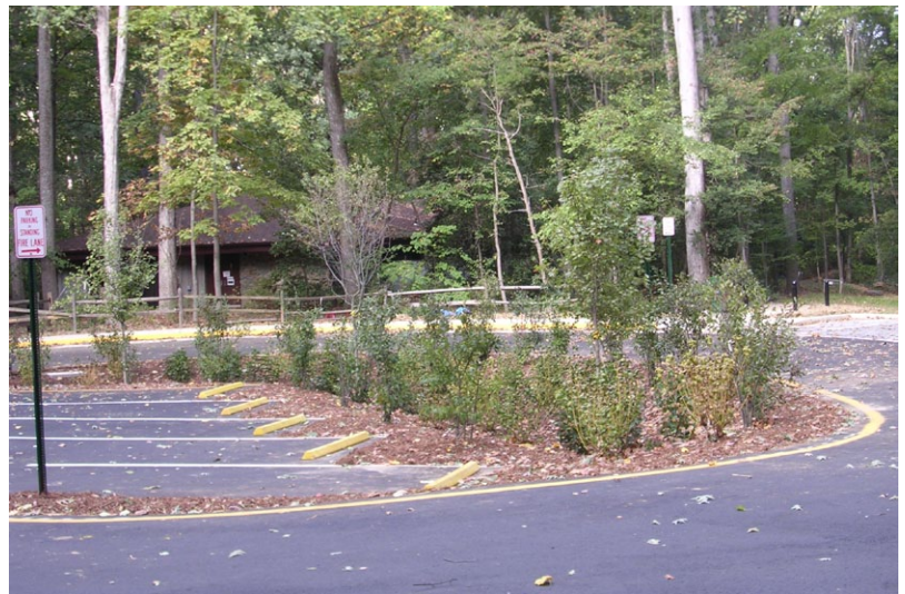
Figure 38: Rain Garden in Parking Lot Example
