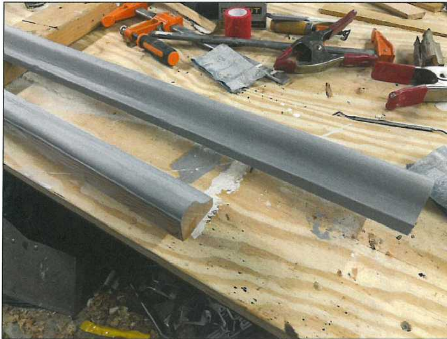
Photo of repair area after coatings applied.
