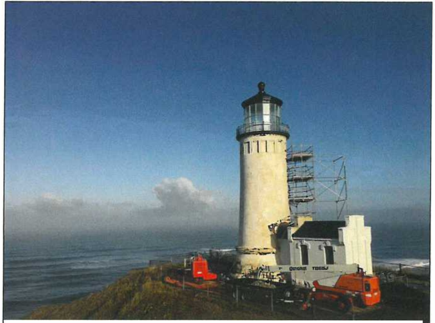
Photo of lighthouse before work commenced.
