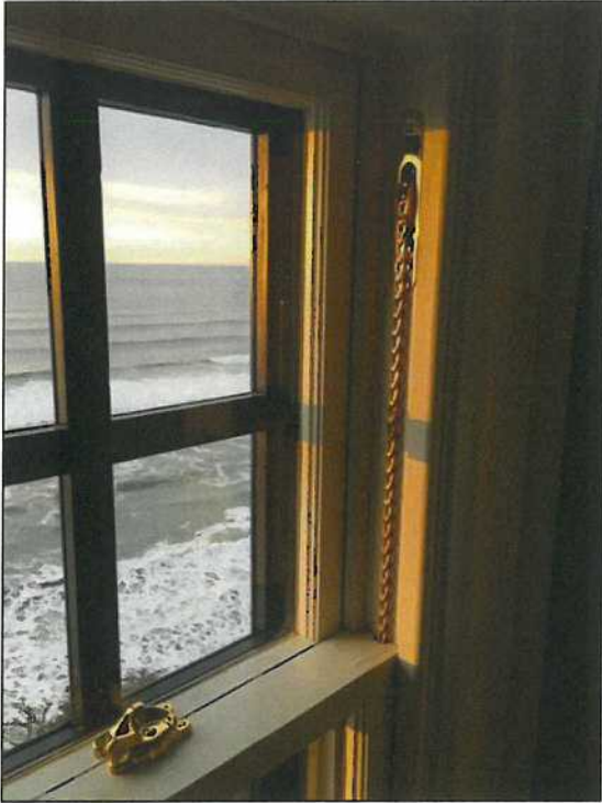
Photo showing new sash and storm window.
