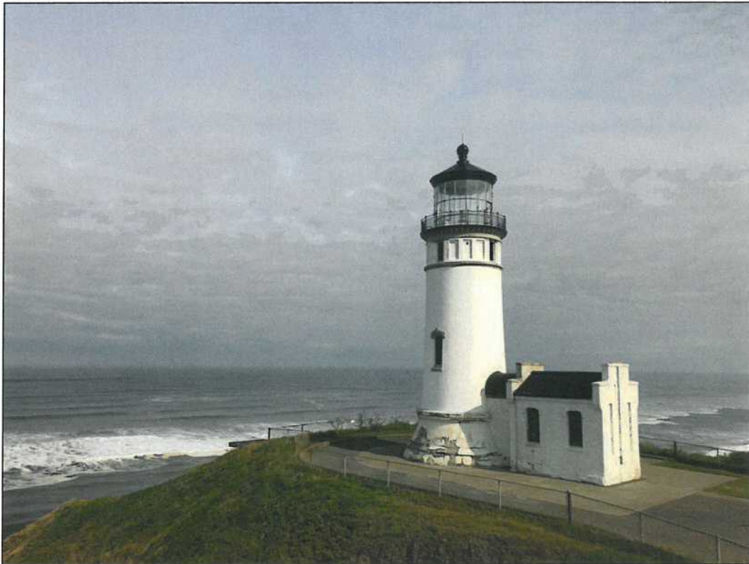
Photo of first phase (Tower Restoration) completed.
