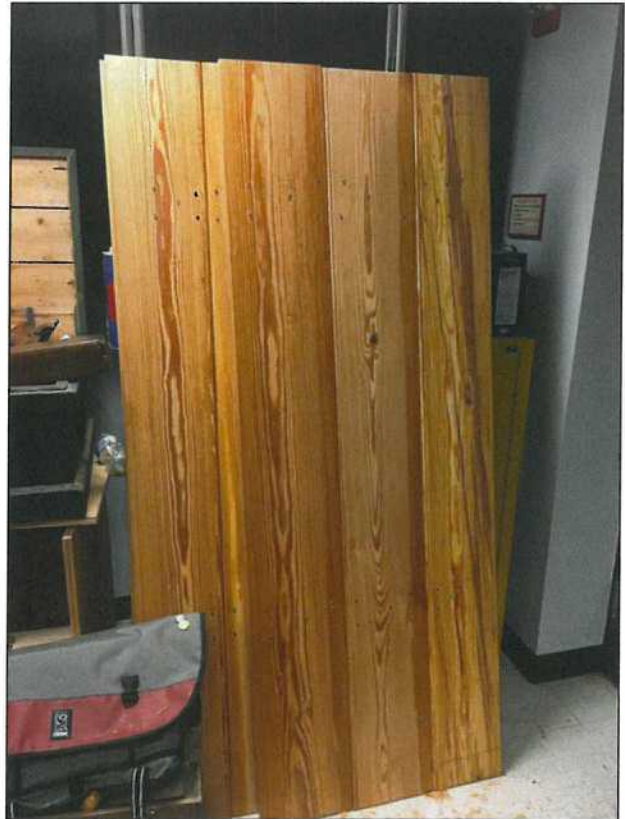
Creation of 4 board and batten doors for the Spinning House.
