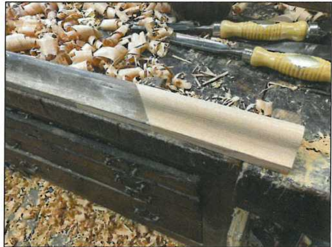
Photo showing infill repair work completed before coatings applied.
