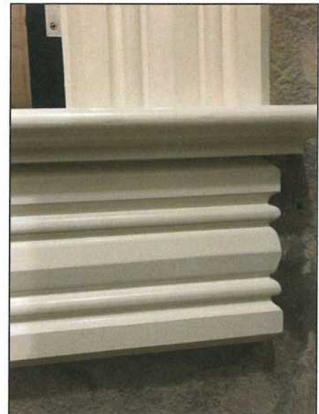
Molding installed in lighthouse.
