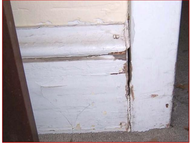
*Image 3.83: Re-nailed Baseboard and Base Molding*
