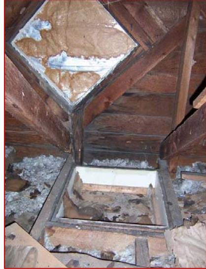
*Image 3.73: Framing for Original Attic Access*
