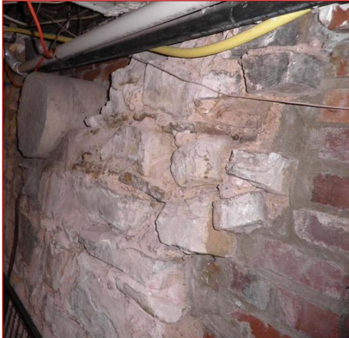
*Image 3.18: Original Foundation Cellar Wall That Has Been Modified*
