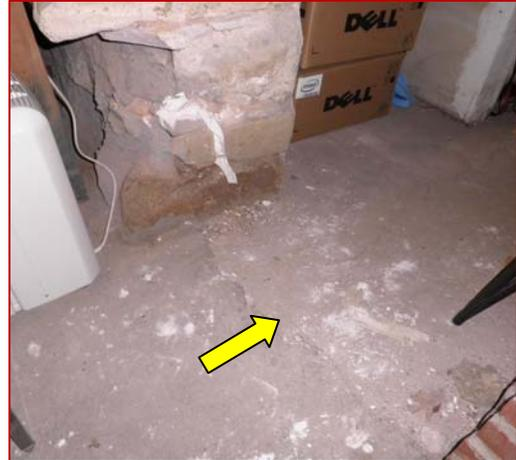
*Image 3.60: Joint of Two Concrete Pours*
