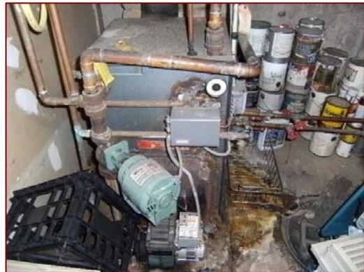
*Image 4.11: Oil-fired Hydronic Boiler*
