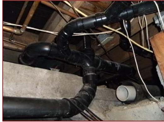
*Image 4.17: Sanitary Sewer Piping*
