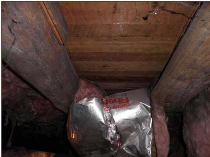
*Image 3.21: Log Joists in Original Portion of House*
