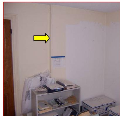
*Image 3.68: Wall Extends Into Bedroom 202 to Increase Original Width of Hallway*
