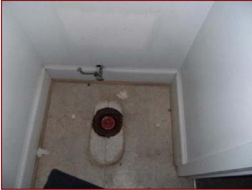
*Image 4.20: Capped Sanitary Sewer Line*
