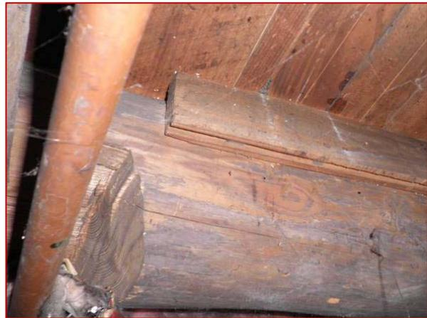
*Image 3.2: Yellow Pine Log First-Floor Joists*
