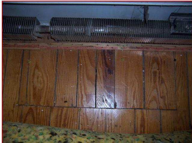
*Image 3.61: Infill at Previous Chimney Flue in Bedroom 201*
