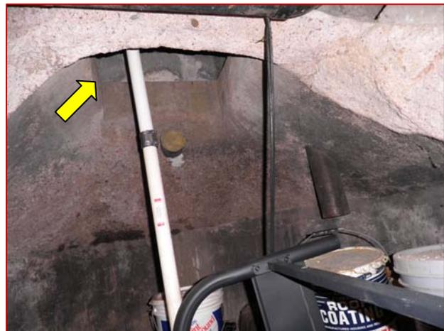
*Image 3.74: Opening at Top of Septic Tank*
