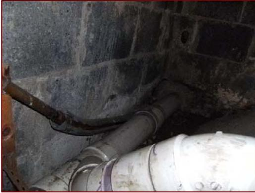
*Image 4.16: Sanitary Sewer Piping*
