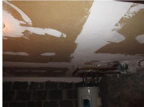
*Figure 70. Drywall compound installation at gypsum ceiling panels in cellar.*
