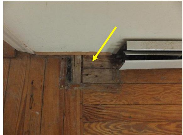
*Figure 84. Exposed wood from pre-existing hallway structural elements. Note intersecting floors.*
