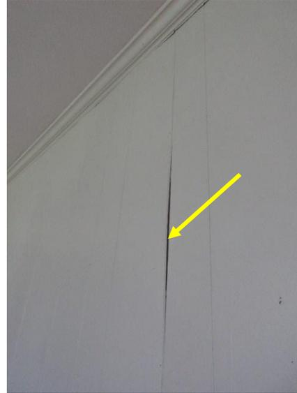
*Figure 66. Displaced wood siding panel, typical.*
