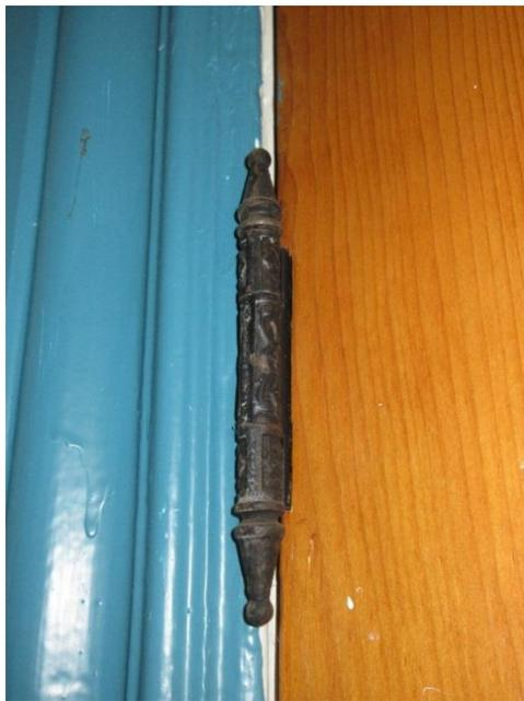
*Figure 95. Original ornate steeple door hinge at D207.*
