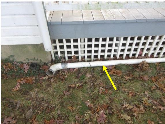
*Figure 35. Disconnected downspout at northwest facade.*
