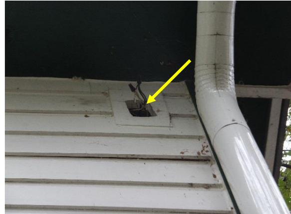
*Figure 44. Missing light fixture at northeast facade.*
