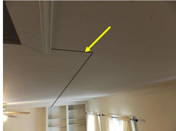
*Figure 46. Cracking at ceiling (1st Floor) likely seams between drywall boards. Cracked traced for clarity.*
