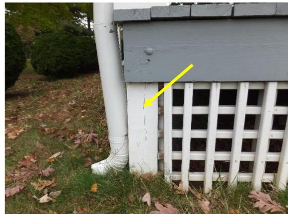
*Figure 36. Vertical separation (checking) at wood porch column.*
