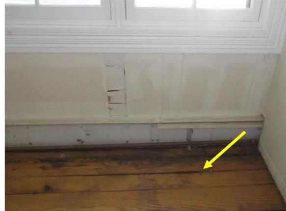
*Figure 86. Staining at wood floor in Room 210 (office). Split across flooring visible.*
