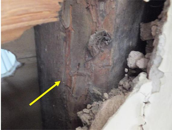
*Figure 55. Original timber framing.*
