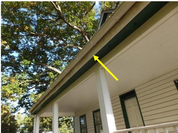
*Figure 31. Soiling at fascia board behind gutter.*
