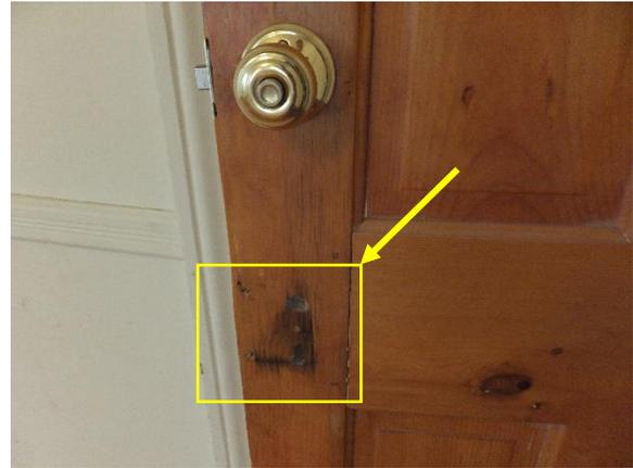
*Figure 94. Missing original rimlock at D101*
