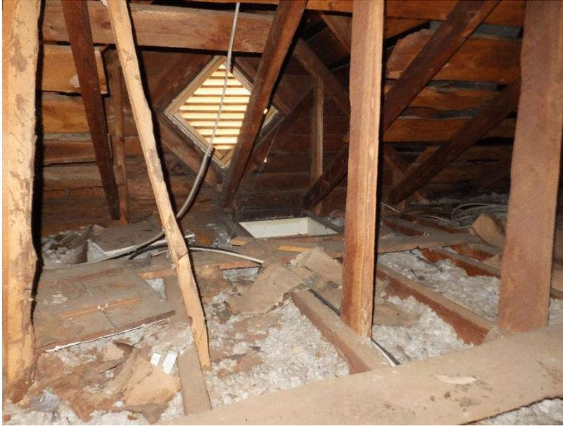
*Figure 2. Framing of original attic access.*
