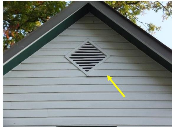
*Figure 12. Example of displaced siding at southwest facade.*
