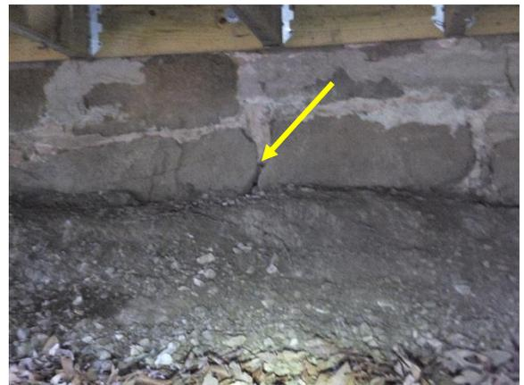
*Figure 40. Missing mortar in stone foundation.*
