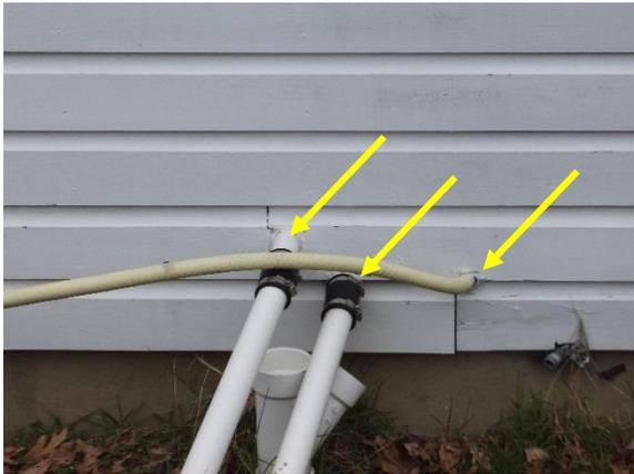
*Figure 25. Partially sealed pipe penetrations on southeast facade.*
