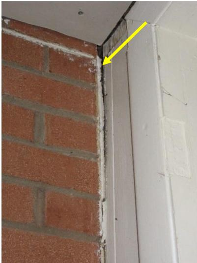
*Figure 83. Separation between brick and adjacent wall, typical.*
