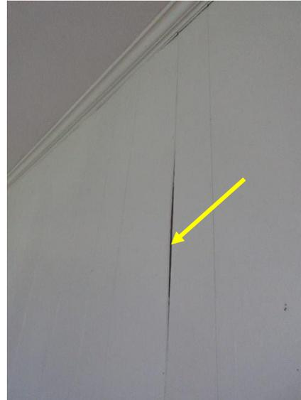
*Figure 66. Displaced wood siding panel, typical.*
