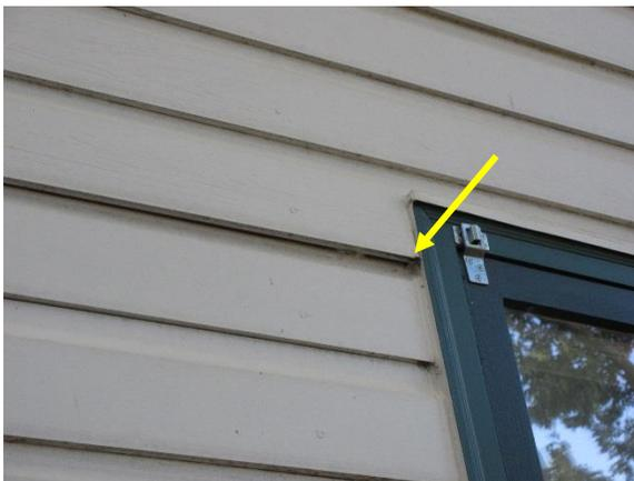
*Figure 13. Displaced wood siding adjacent to window a northwest facade.*
