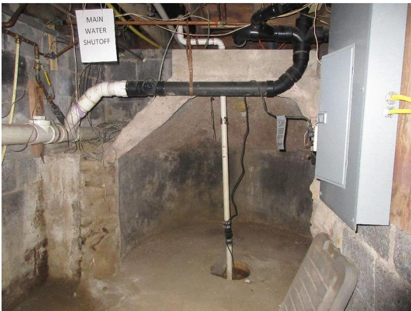
*Figure 3. Original septic tank exposed in cellar.*
