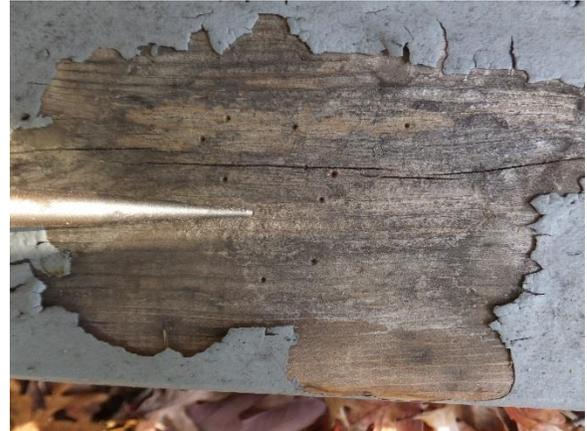
*Figure 38. Paint and wood deterioration at porch stairs.*
