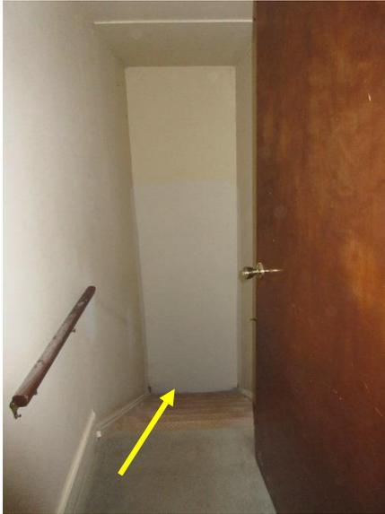
*Figure 69. Terminated exterior access of stairwell at D205.*
