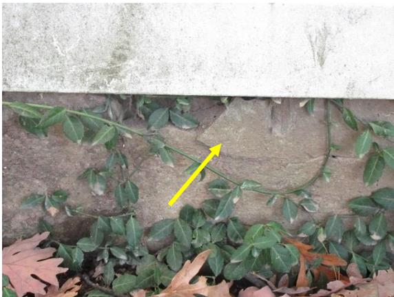
*Figure 21. Incipient spall in parge coat at original foundation near window well.*
