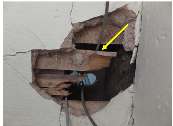
*Figure 54. Hole through plaster and lathe for wiring.*
