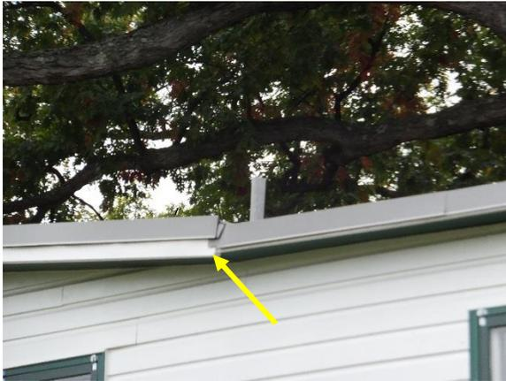
*Figure 33. Displaced roof coping on southeast facade.*
