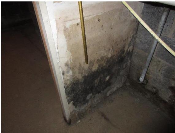
*Figure 71. Potential microbial growth at drywall in cellar.*
