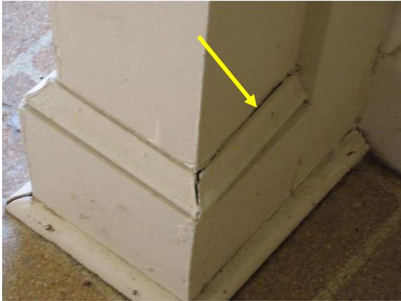
*Figure 61. Gap and separation at crown molding, typical.*
