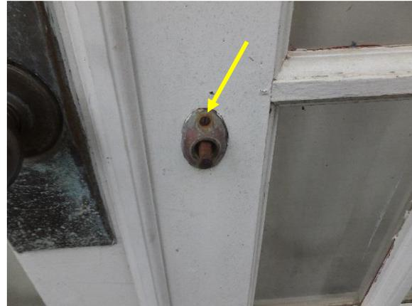
*Figure 30. Missing doorknob at French doors on northeast facade.*
