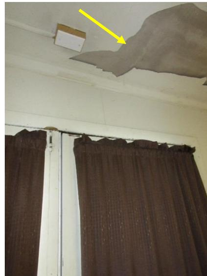
*Figure 58. Drywall delamination at rear entryway.*
