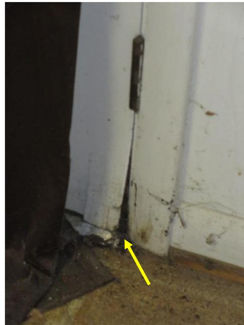
*Figure 96. Damage at the trim of the French Doors.*
