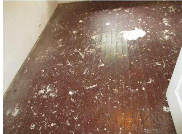
*Figure 92. Typical brown painted wood floor with white splattered paint.*
