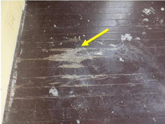
*Figure 93. Paint scraped from wood floor.*
