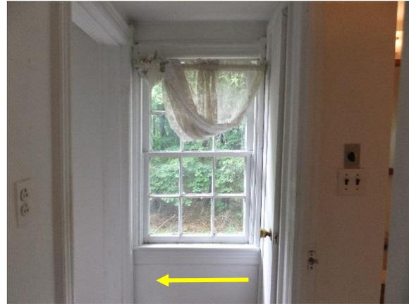
*Figure 37. Window 204 sloped to the west.*
