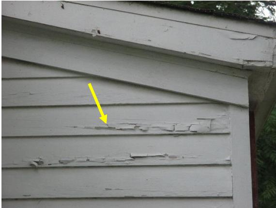
*Figure 16. Typical paint deterioration on wood siding.*
