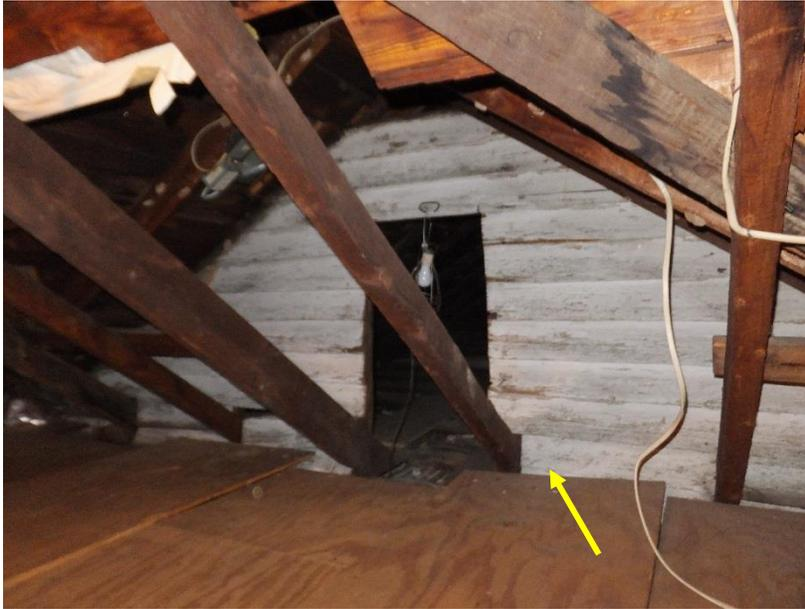
*Figure 7. Previously exterior west gable of the Period I section of the home as viewed from the Period II attic space.*
