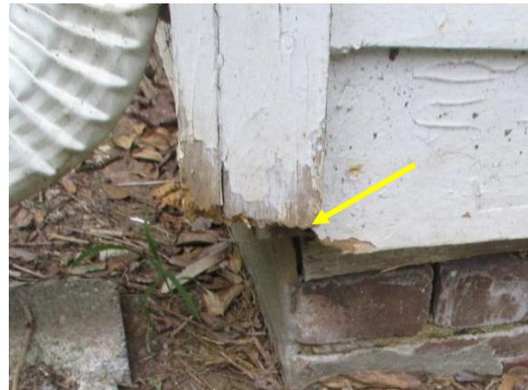
*Figure 11. Deteriorated wood at trim element on corner. Note exposed brick at foundation where parge coat and brick mortar are no longer intact.*
