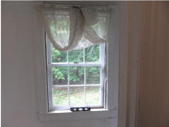
*Figure 38. Window 205 sloped to the east.*
