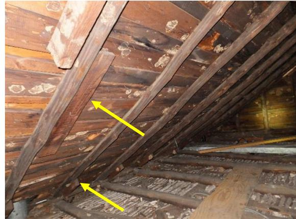
*Figure 86. Peeled log rafters in attic with additional milled lumber for decking.*
