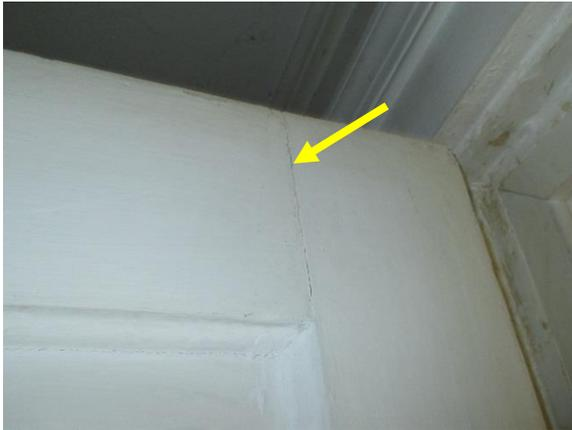
*Figure 95. Typical separation of joinery at historic interior doors.*
