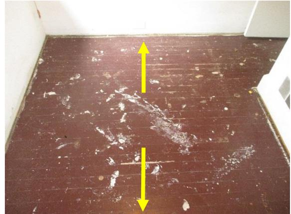
*Figure 94. Sloped floor in room 202.*
