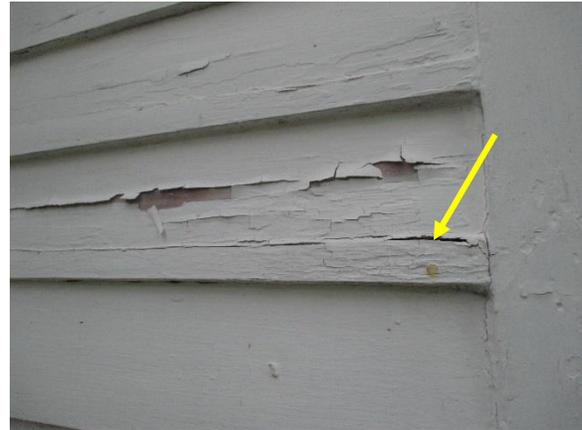
*Figure 21. Split in wood originating from edge of wood board above fastener.*
