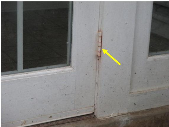
*Figure 34. Corroded hinges at southwest french doors, typical condition for exterior doors on the home.*
