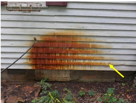
*Figure 18. Ferrrous staining on east facade adjacent to water spigot.*
