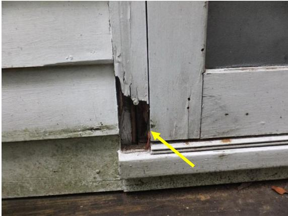
*Figure 32. Missing section of wood at the base of an east screen door.*
