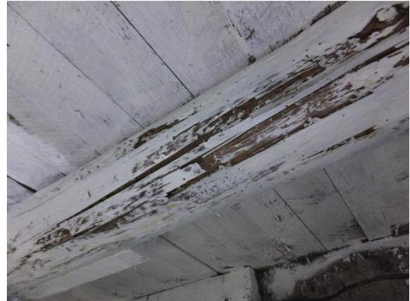
*Figure 74. Soft and splintered 3/4 round beams in cellar.*
