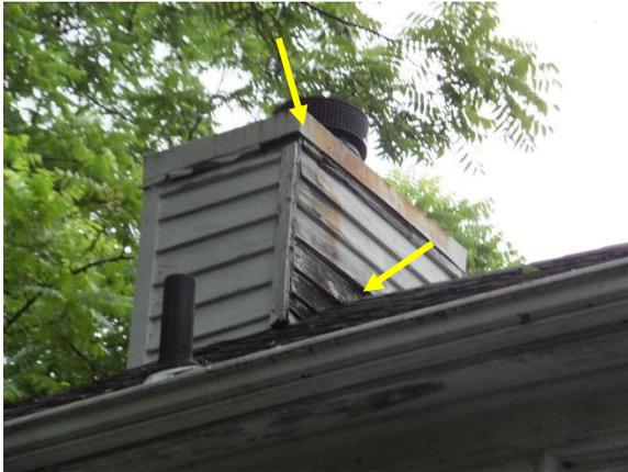
*Figure 28. Dark and ferrous staining at the chimney.*
