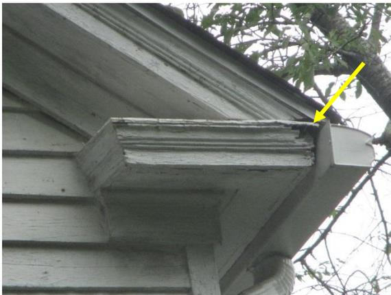
*Figure 12. Deteriorated wood at cornice element on northwest corner behind gutter.*
