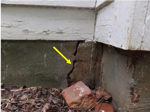
*Figure 26. Crack and delamination in parge coat that covers brick foundations.*
