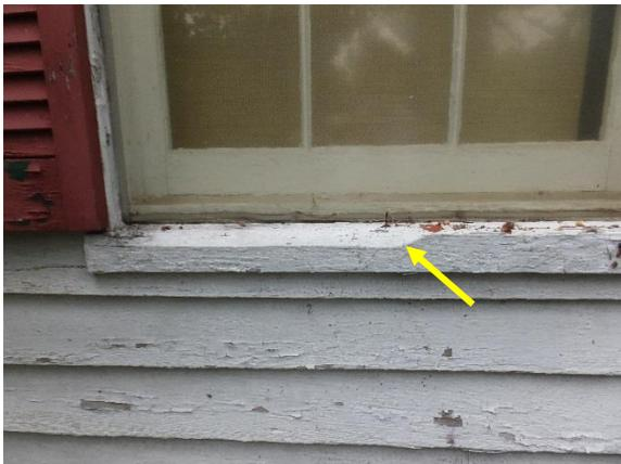
*Figure 46. Area of missing wood at a first floor window sill on west facade.*
