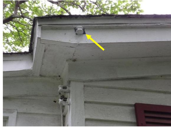
*Figure 25. Rough opening through the cornice for the utility line anchor.*
