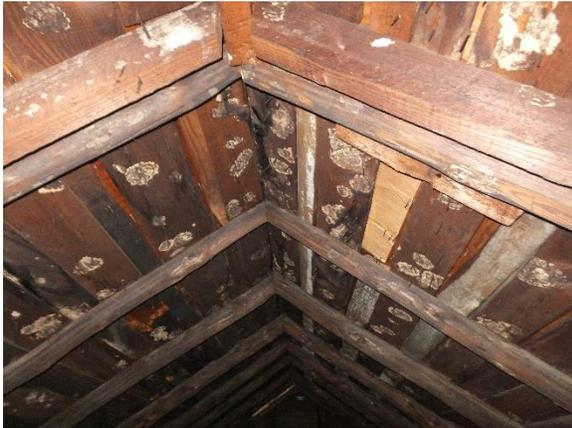
*Figure 87. Historic peeled log rafters toe-nailed without a ridge beam or board in attic.*
