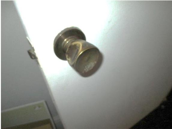
*Figure 99. Crushed door knob at door D115.*
