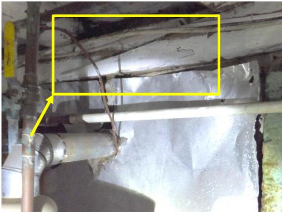
*Figure 77. Full-depth split through timber sill in cellar.*
