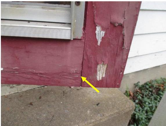
*Figure 30. Typical separation of joinery at doors.*
