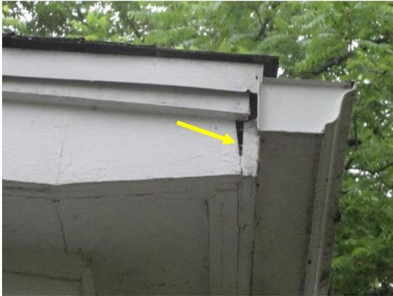
*Figure 24. Separation of wood fascia board adjacent to the gutter.*
