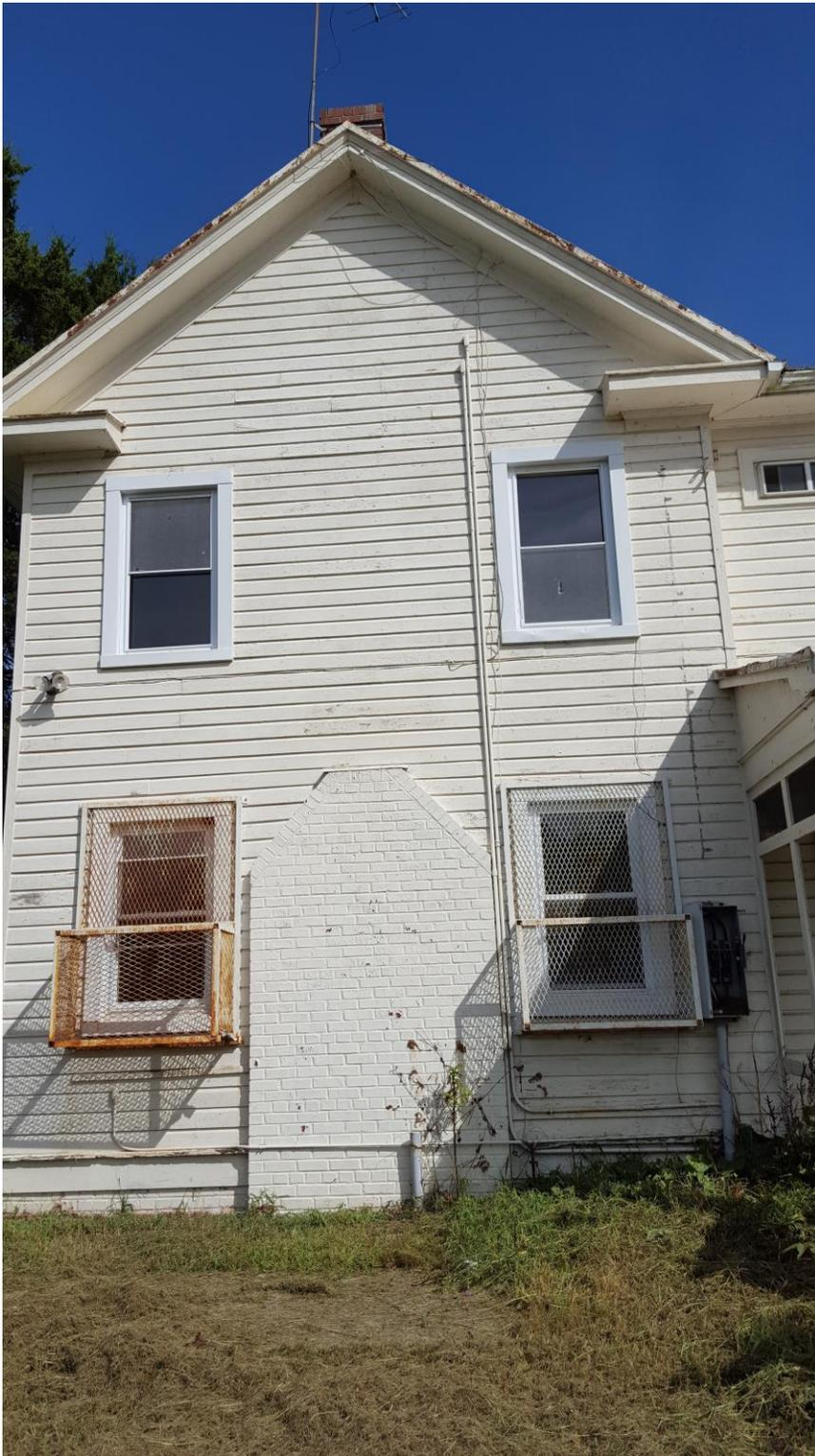
*Side Elevation with masonry chimney*
