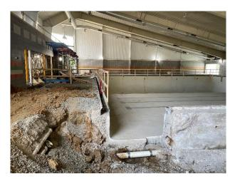
The majority of construction to date has consisted of demolition of portions of the existing structure. Many existing interior walls have been removed, and portions of the slab have been cut to accommodate drain lines for the relocated and expanded locker rooms. There is extensive demolition around the pool area to facilitate updated drainage and mechanical systems.
