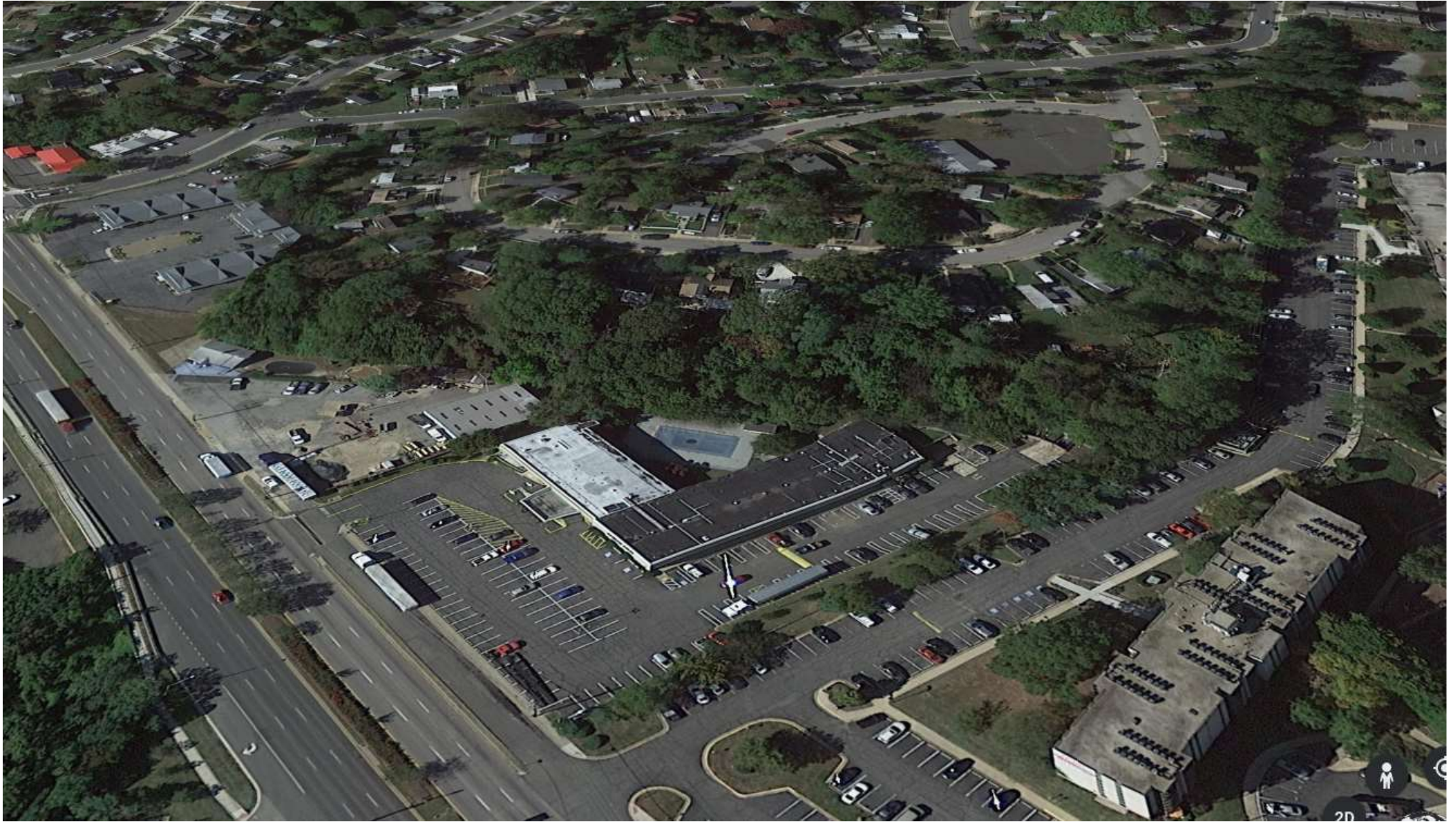
Existing Conditions - 6100 Richmond Highway Looking Southwest
