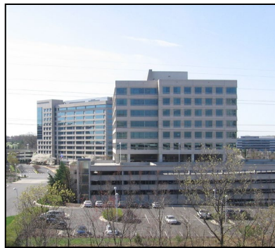
Two Discovery Square, a medium intensity office building and parking garage located in Reston Town Center.
