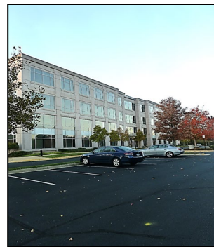
Arboretum building, a low intensity office building near the Sunrise Valley Wetlands.
