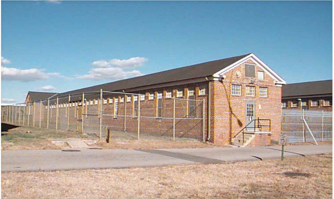
Dormitory at the Central Facility
