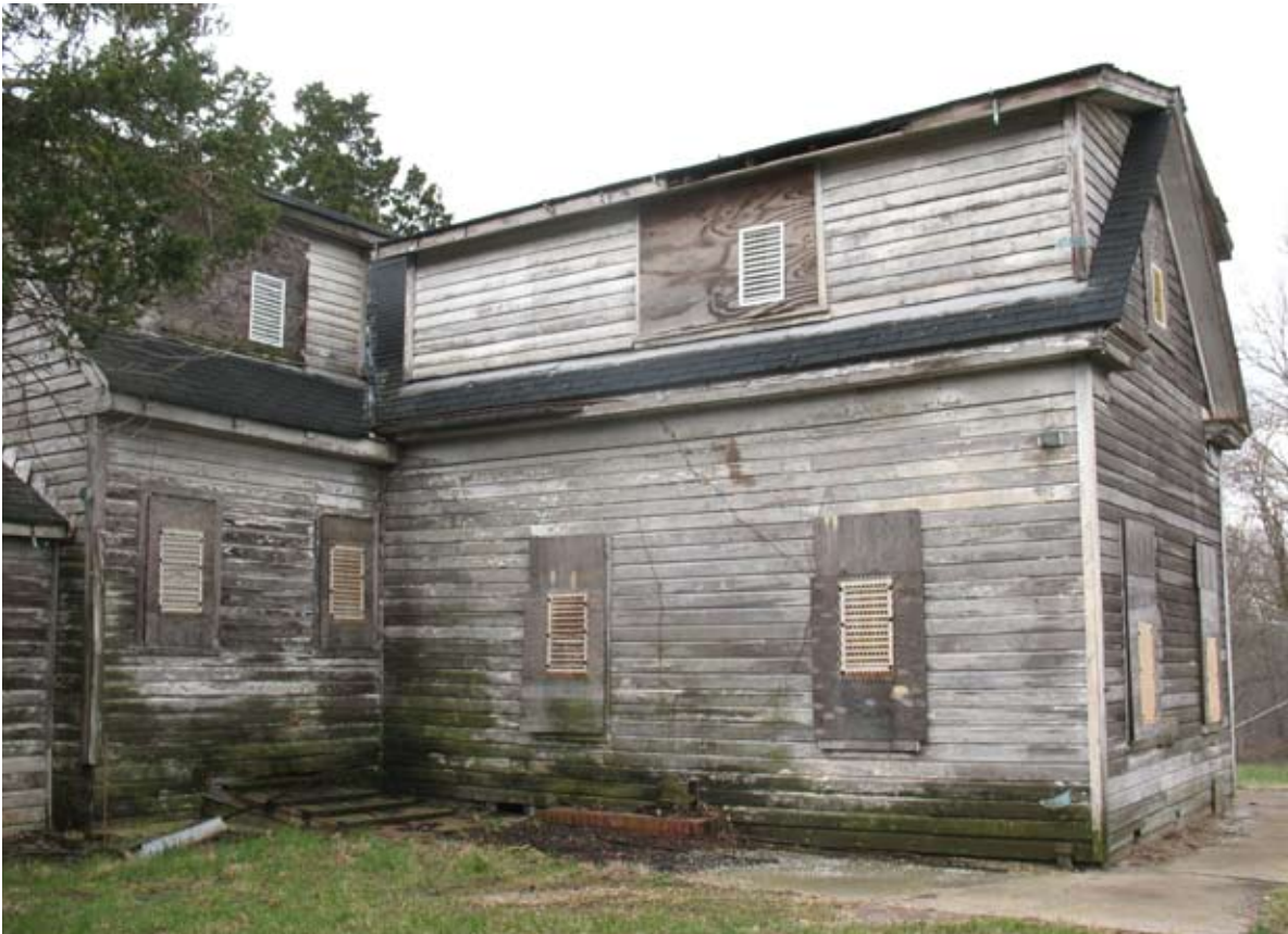
Laurel Hill House – April 2011 view from northeast. Note moisture saturation of wood siding at base.
