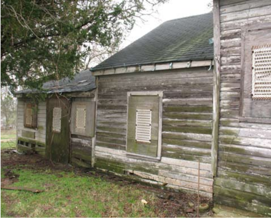
Laurel Hill House – April 2011 view from north side. Note poor condition of roof above entrance.
