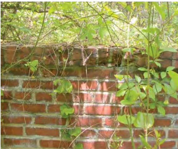
Figure 3-52. Cracking on the south side of the central wall coping.
