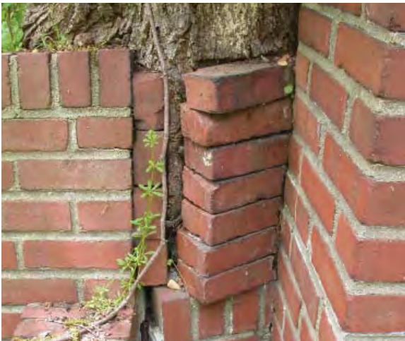
Figure 3-45. Tree growth has caused a major displacement of the wall adjacent to the brick bench.
