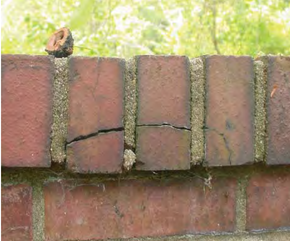
Figure 5-10. Typical cracking occurring along wall copings.
