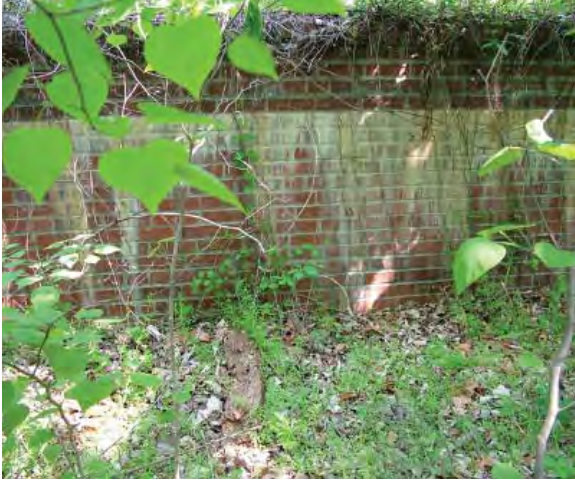
Figure 3-50. The central retaining wall, ninety-five feet in length, is aligned on the cross-axis of the Terraced Garden. Note efflorescence.
