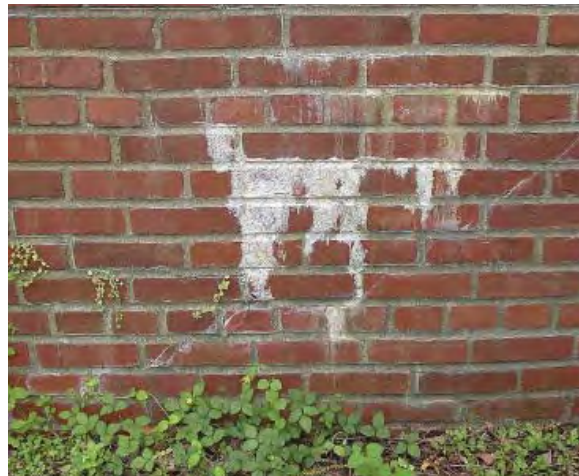
Figure 5-6. Typical efflorescence on face of retaining walls.
