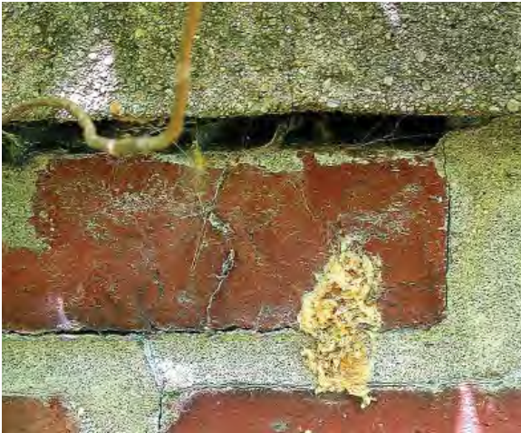
Figure 5-11. Typical example of mortar missing from brick joint.
