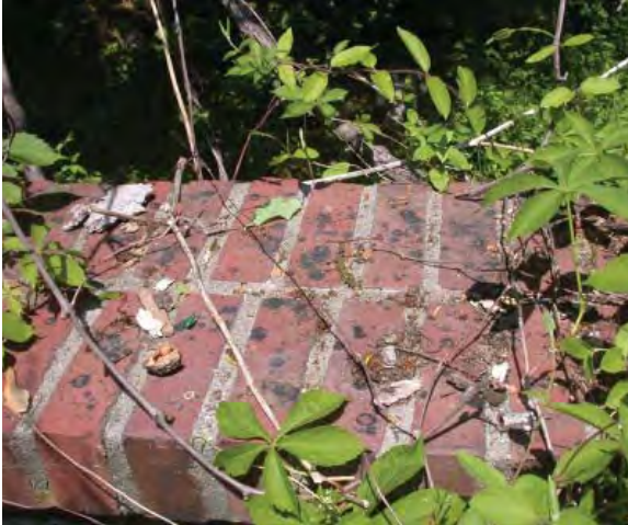
Figure 3-53. Dark staining is evident on top of the coping on the semi-circular terrace retaining wall.
