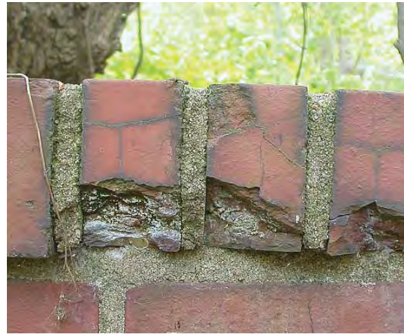
Figure 5-9. Example of spalling condition of some brick.
