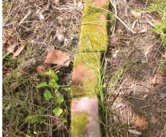
Figure 5-5. Typical biological growth on planting border brick.
