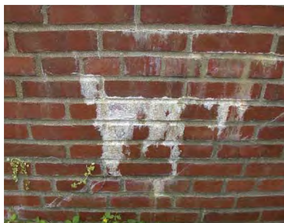
Figure 3-25. Efflorescence along the west inside cheek wall of the steps of the west entrance stairway.
