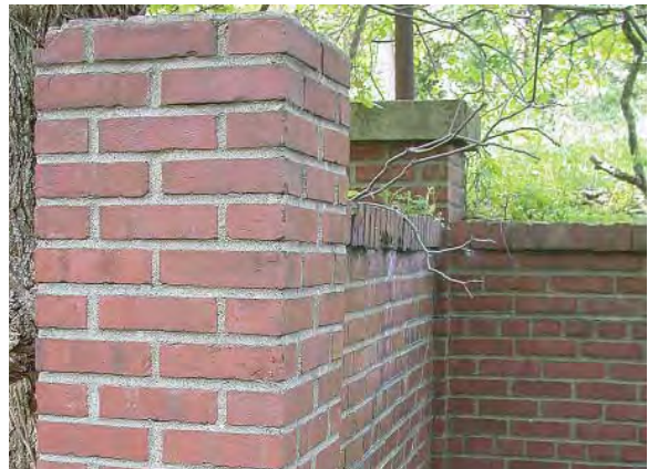
Figure 5-13. The capstone element is missing from this section of wall.
