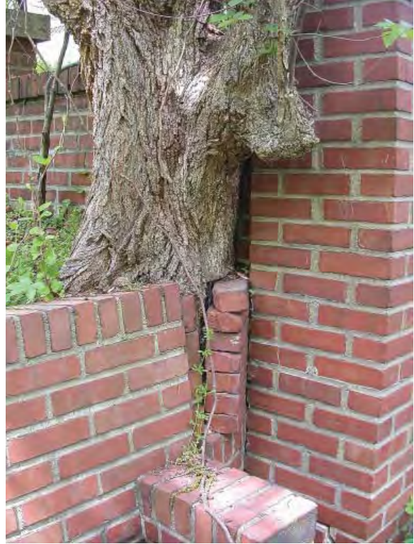
Figure 5-12. Displacement of masonry at infill between bench and bench stair wall.
