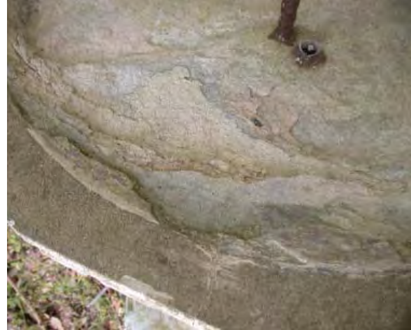
Figure 5-8. Delamination occurring in fountain basin.
