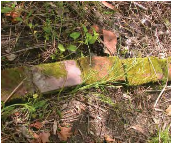
Figure 3-66. Most of the Terraced Garden's planting beds and paths are edged with bricks that are accumulated with soil and biological growth.
