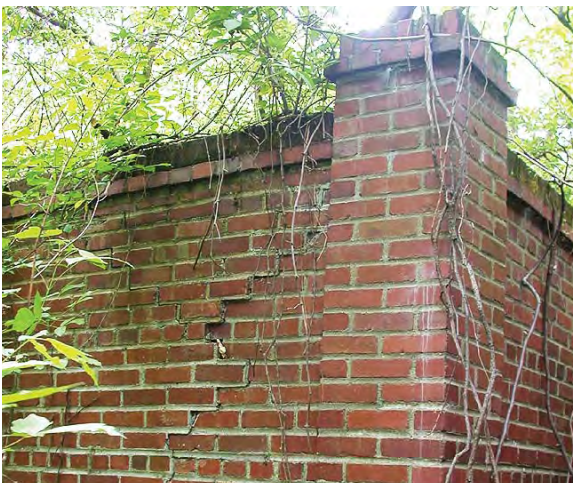
Figure 3-55. The east terrace retaining wall has a significant crack due to differential movement of the wall and rock garden stairway.
