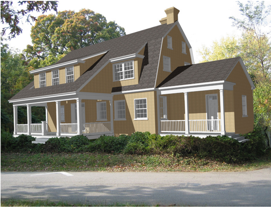
Figure 2.5 This photo-simulation shows the appearance of the south elevation after the stucco had been applied to the exterior and before the office door was replaced and the front porch screened.
