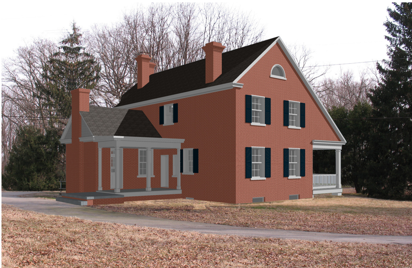
Figure 2.4 This photo-simulation of the rear of the Physician's Residence represents the appearance of the brick house with shutters, which were likely removed when the stucco was added. Also note that there was likely some type of a gable roof over the kitchen, approximating this wing's appearance before the sunroom was added.
