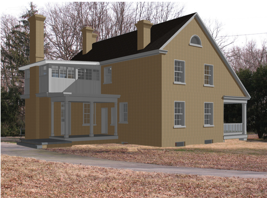
Figure 2.6 In this photo-simulation of the rear of the house, the shutters have been removed and the sunroom added over the kitchen.
