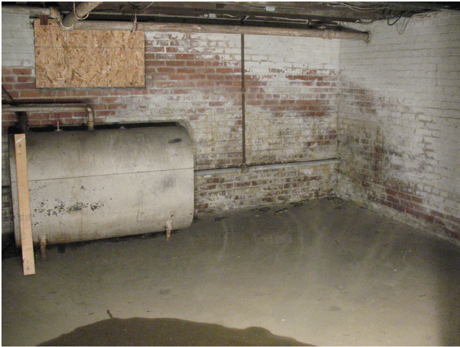
Figure 3.47 Room 004 is located under the east side of the house and is a mechanical space with a concrete floor and painted brick walls.
