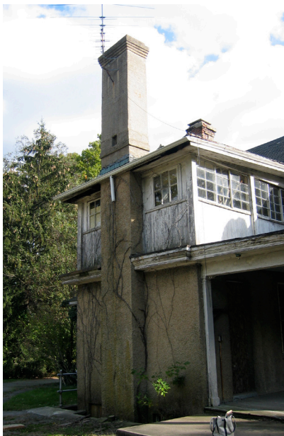
Figure 3.30 The kitchen chimney features a band above the sunroom roof line that shows where the chimney was extended after that addition.
