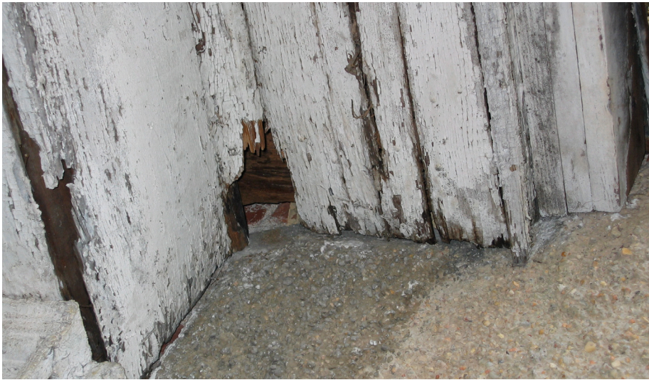
Figure 3.23 This view shows the original brick beneath stucco and that the stucco stops at the wood trim, and that therefore the stucco was a later addition.
