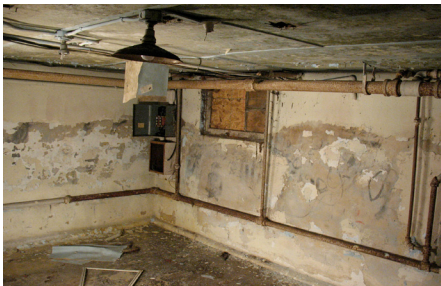
Figure 3.71 Room 001 has parged walls and mold growth on the ceiling.
