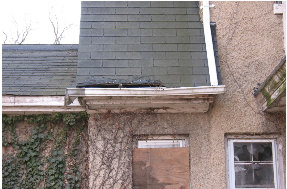
Figure 3.42 Water damage has occurred on the eave of the north elevation, east of the sunroom addition.
