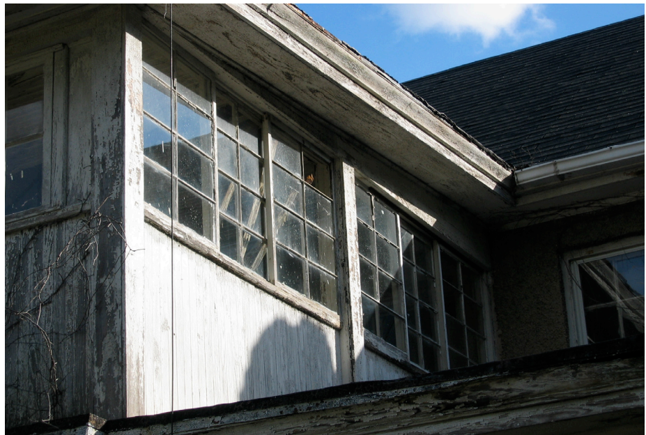
Figure 3.25 This view of the west elevation of the sunroom addition shows its frame construction.
