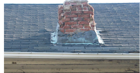
Figure 3.31 The deteriorated condition and reduced height of the living room chimney are clearly visible.
