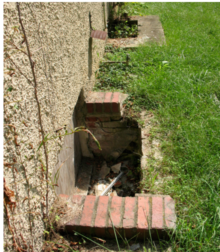
Figure 3.39 Concrete and masonry window wells are located on the west elevation.
