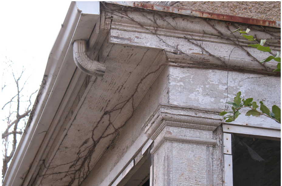
Figure 3.43 The ogee-shaped gutter and missing downspout are shown here on a corner of the front porch.
