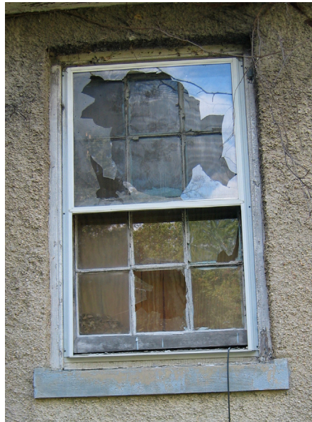
Figure 3.37 Broken panes and bare wood are evidence of the deteriorated condition of the house's wooden windows and damage to the existing storm windows.
