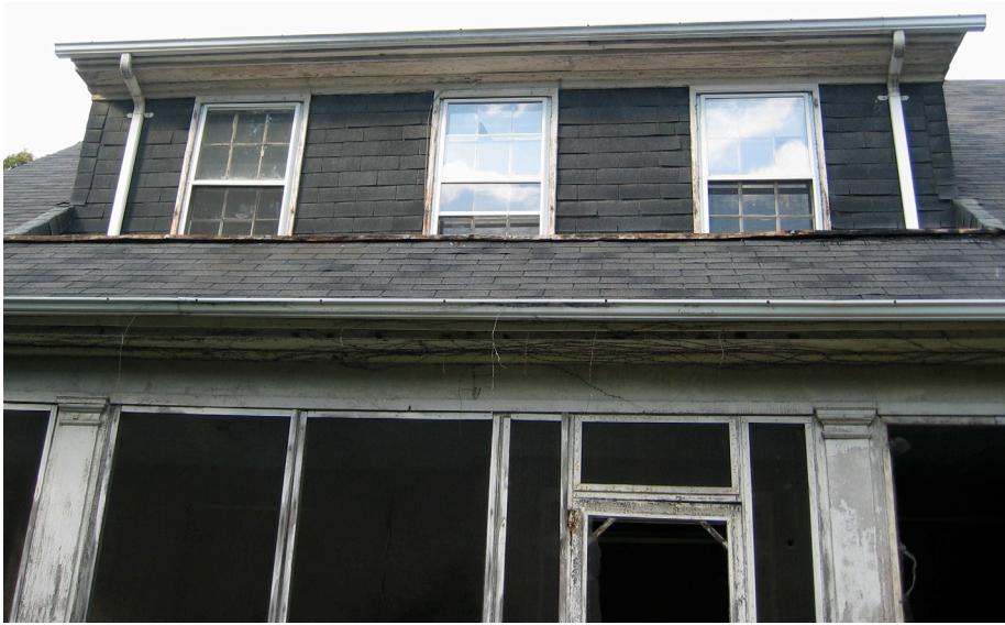
Figure 3.44 The shed dormer is located within the main roof on the south elevation.
