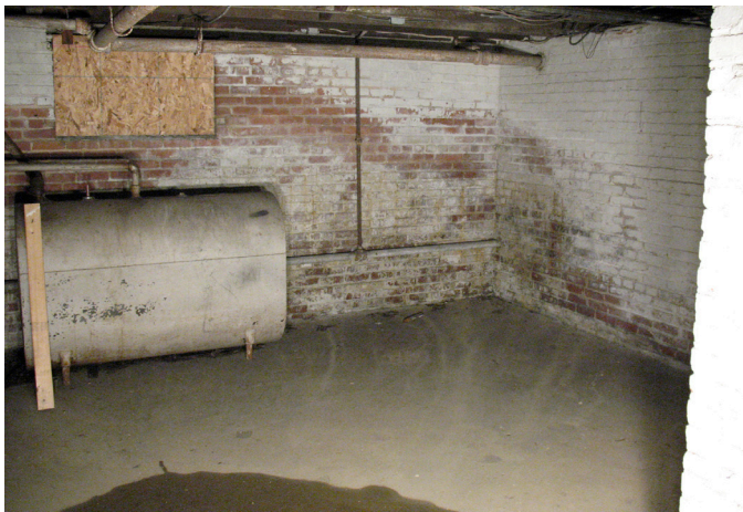
Figure 3.68 There is a poured concrete floor in the basement.
