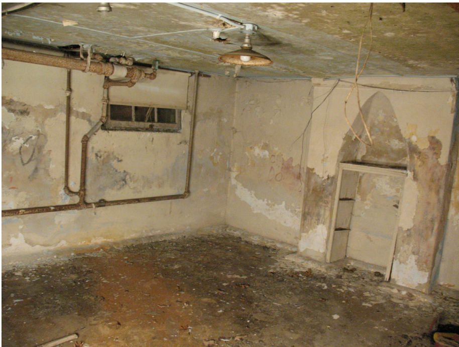
Figure 3.49 Room 001 occupies the west side of the basement and has a plaster coat over the brick foundation walls.
