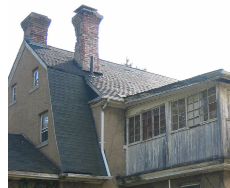
Figure 3.32 The failure of the stucco coat on the chimneys on the north side of the house is evident.
