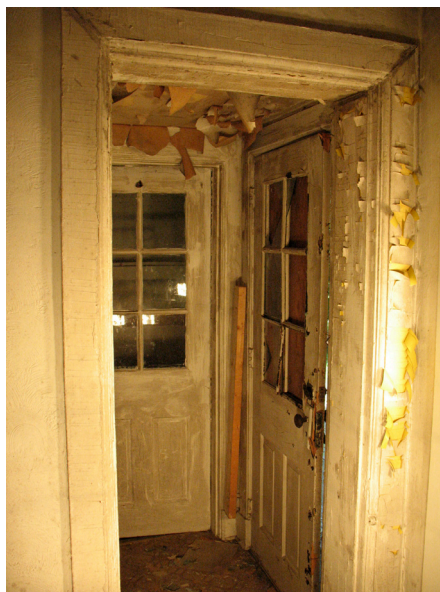
Figure 3.76 A six-light interior door is located between Rooms 103 and 105.
