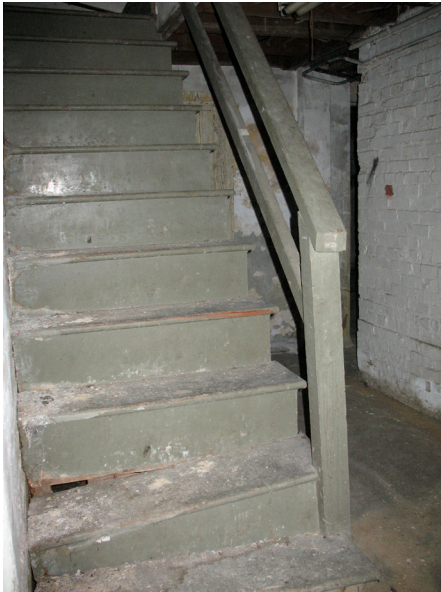
Figure 3.63 The collapsing tread and riser are evidence of the deteriorated condition of the basement stairway.
