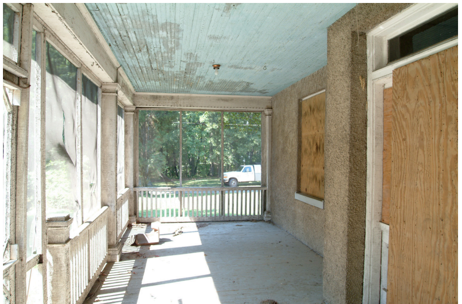
Figure 3.28 The screened front porch exhibits deteriorated wood finishes.
