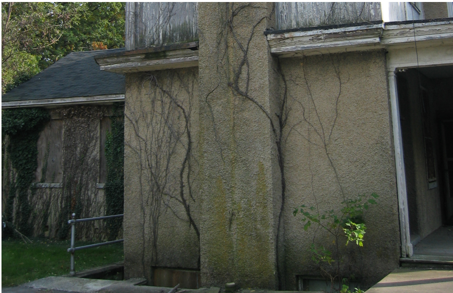
Figure 3.24 Vine growth and moss are evident on the north wall of the kitchen wing.
