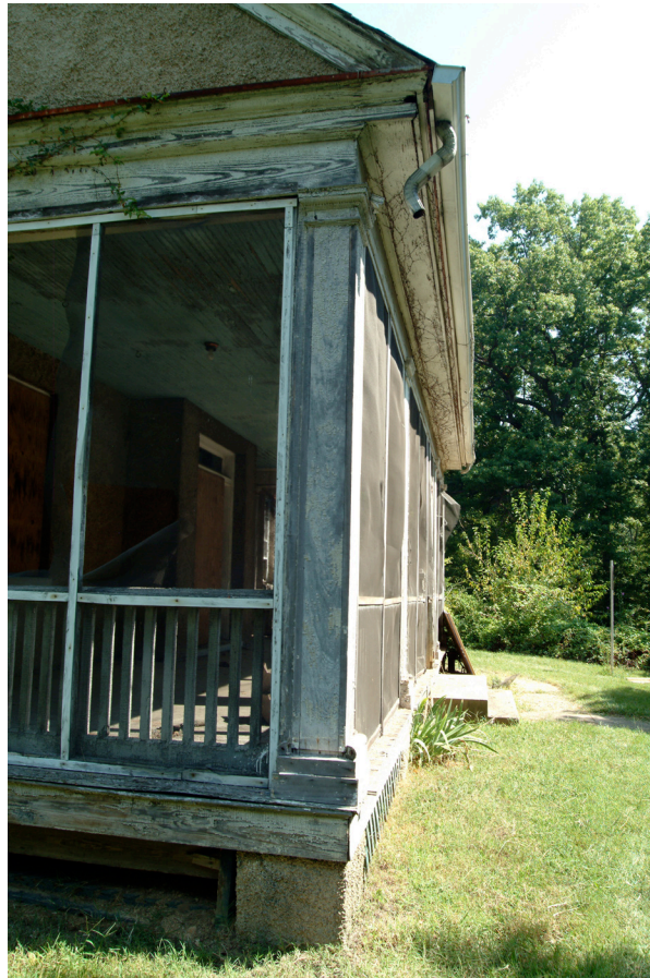
Figure 3.22 Stucco-covered brick piers provide the foundation for the front porch.
