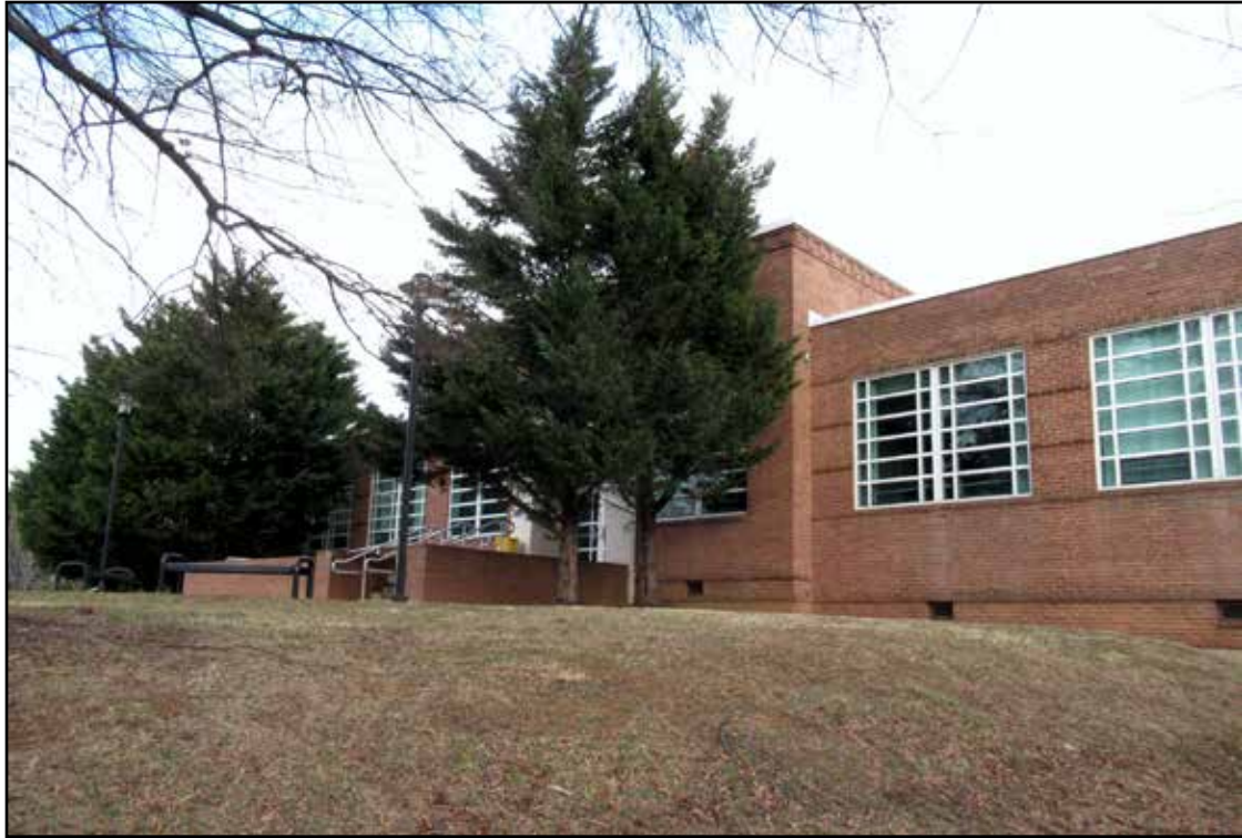
Figure 3.64. James Lee Community Center (029-6030), original facade.
