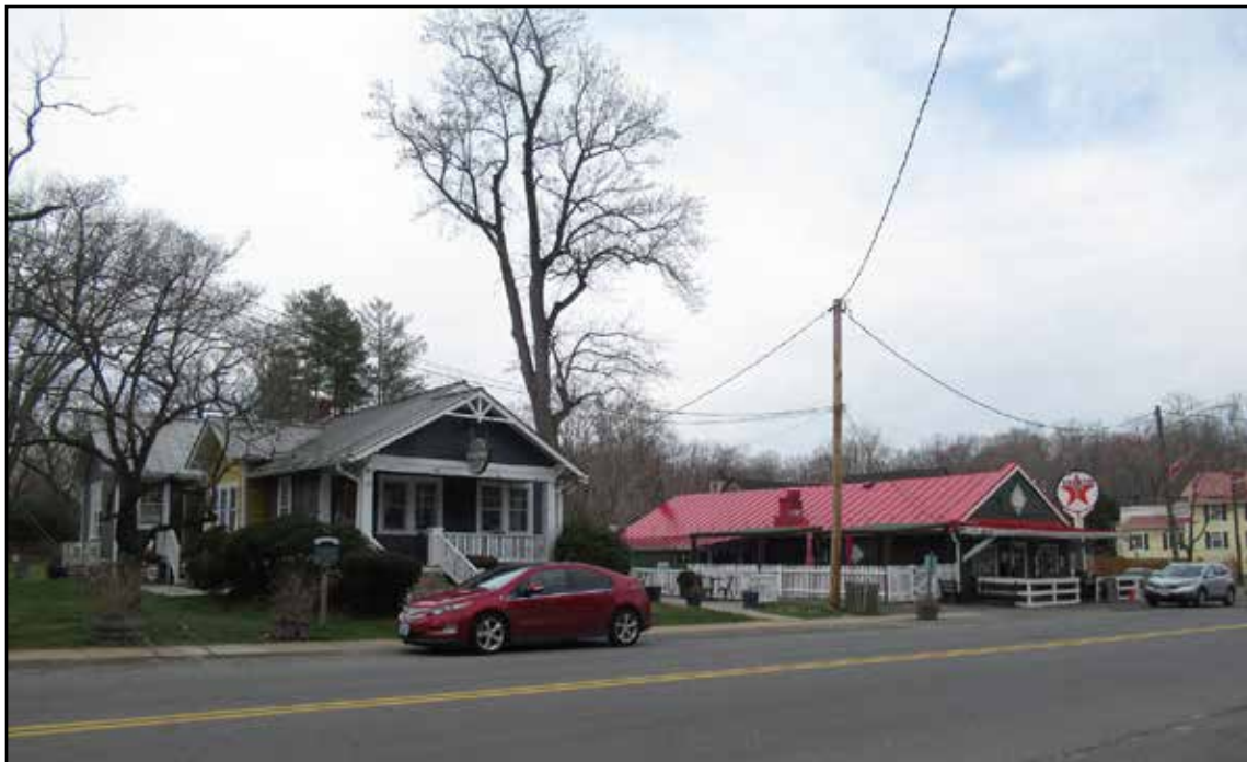
Figure 3.27. Clifton Historic District (194-0003), Main Street, view to northwest.
