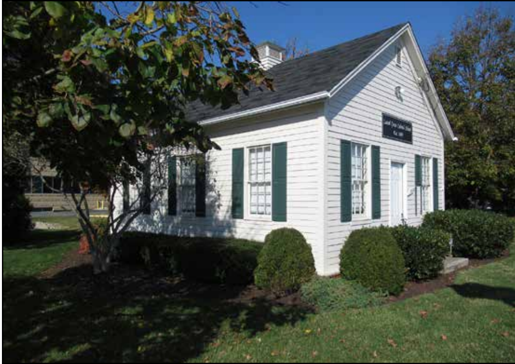
Figure 3.70. Laurel Grove School (029-0361), southeast corner.
