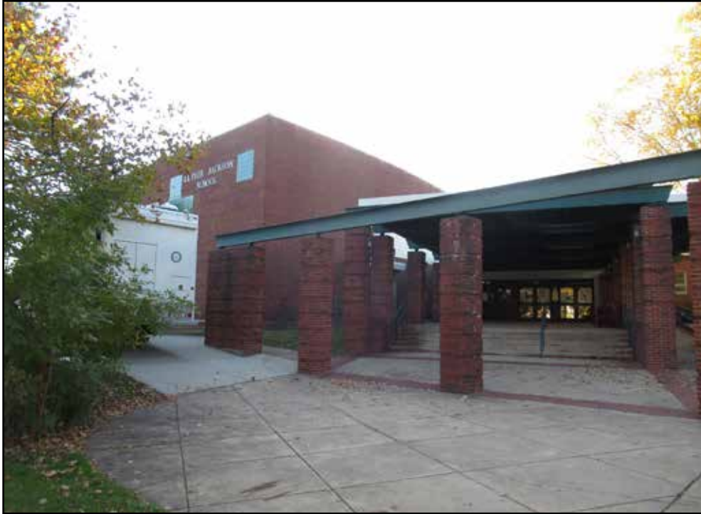
Figure 3.81. Luther P. Jackson School (029-5318), east elevation, view to southwest.
