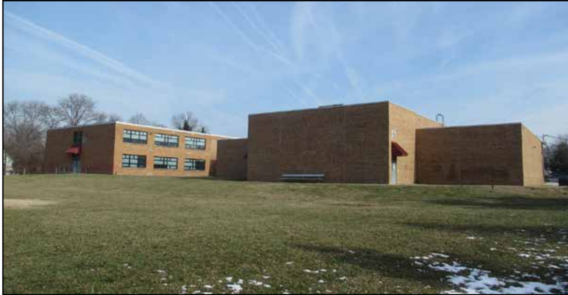
Figure 3.104. Quander Road School (029-6908), southwest corner.
