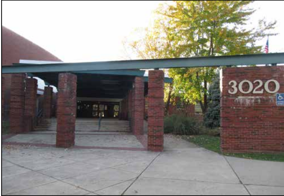
Figure 3.83. Luther P. Jackson School (029-5318), primary entrance.
