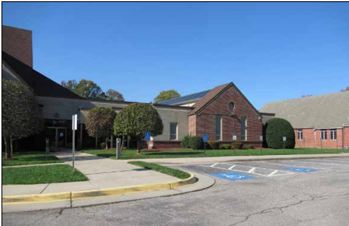
Figure 3.9. Bethlehem Baptist Church (29-6007), new church, north wing facade.
