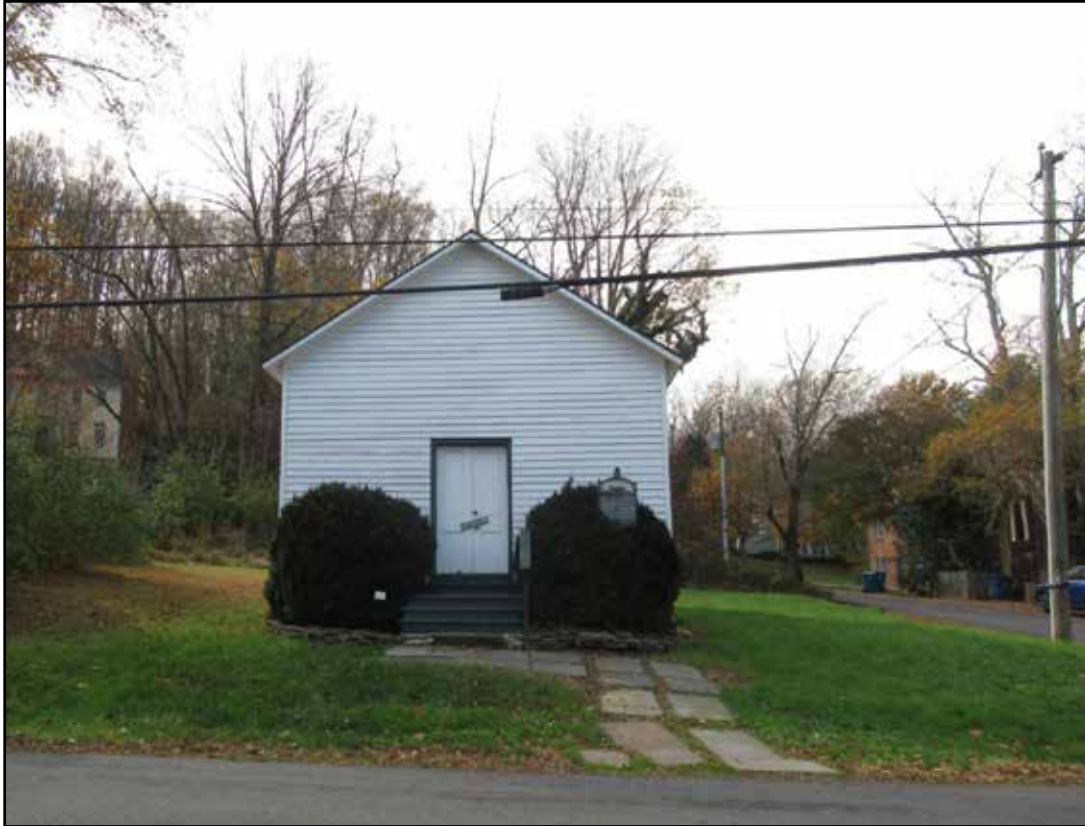
Figure 3.29. Clifton Primitive Baptist Church (194-0003-0024), facade.
