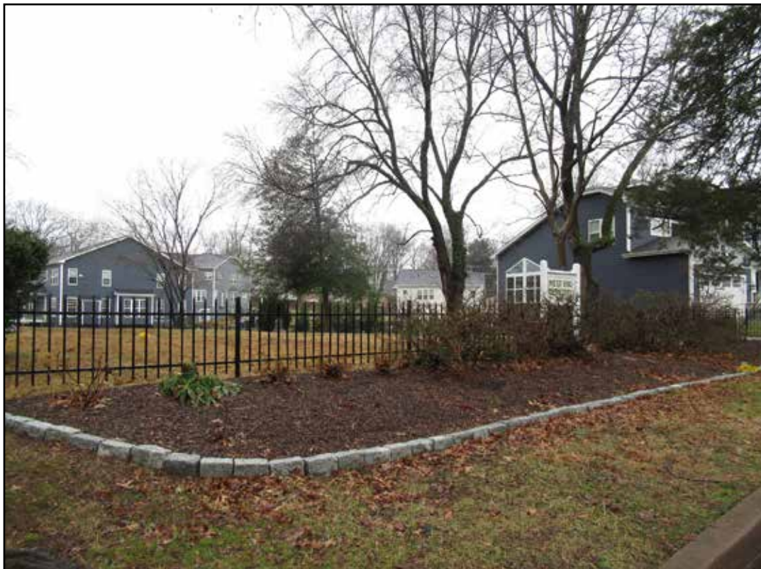
Figure 3.139. West End Cemetery (153-5019), view to the northwest.
