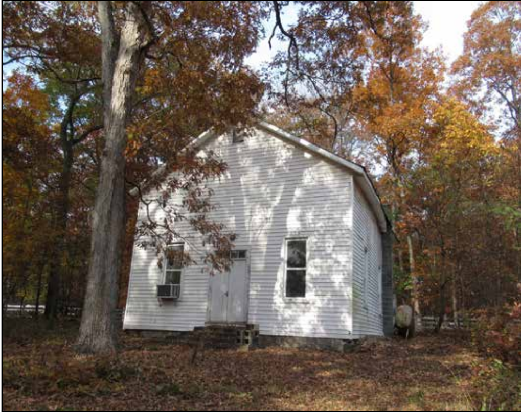
Figure 3.40. Cub Run Primitive Baptist Church (029-5321), facade.
