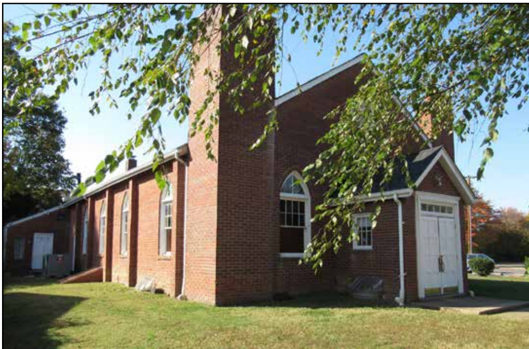
Figure 3.141. Woodlawn Methodist Church (029-6045), southeast corner.
