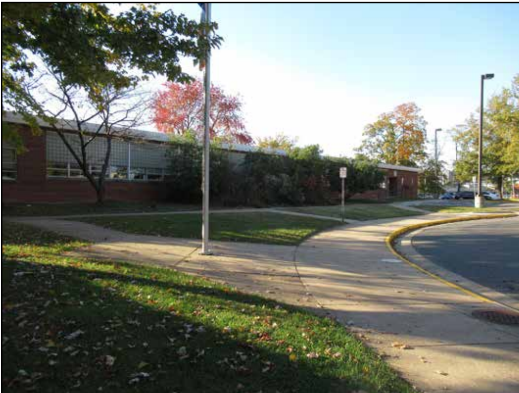
Figure 3.82. Luther P. Jackson School (029-5318), east elevation, view to northwest.
