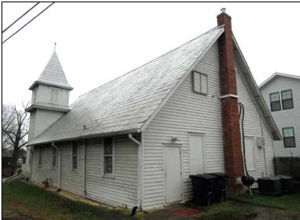
Figure 3.46. First Baptist Church of Vienna (153-5017), west corner.
