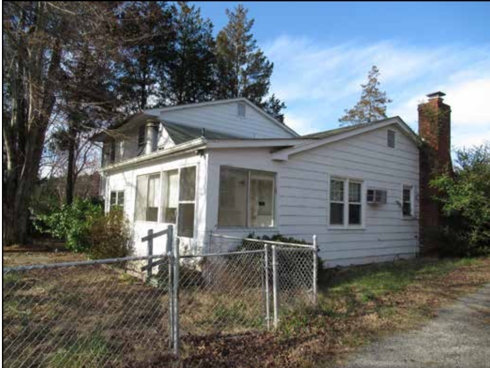
Figure 3.10. Bushrod House (029-6929), south corner.
