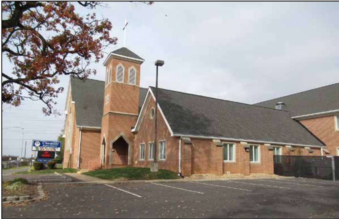
Figure 3.17. Chantilly Baptist Church (029-0307), east elevation.
