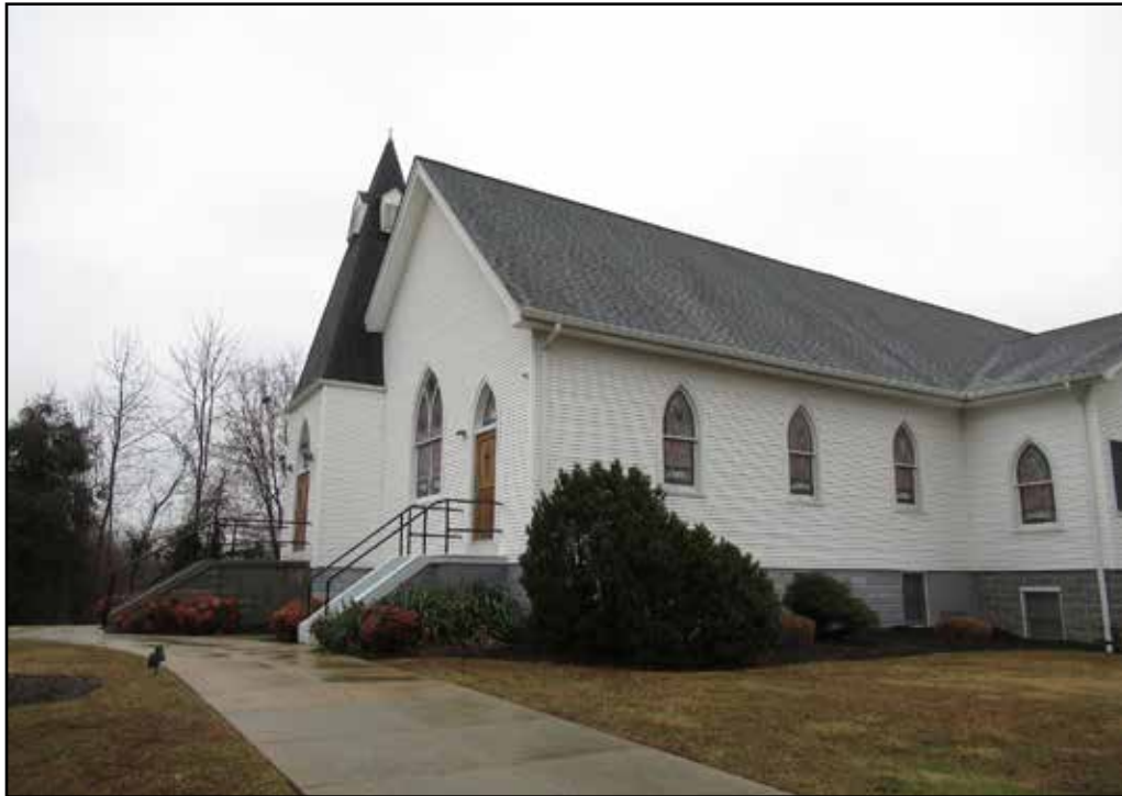
Figure 3.115. Shiloh Baptist Church of Odrick's Corner (029-0189), southwest corner.
