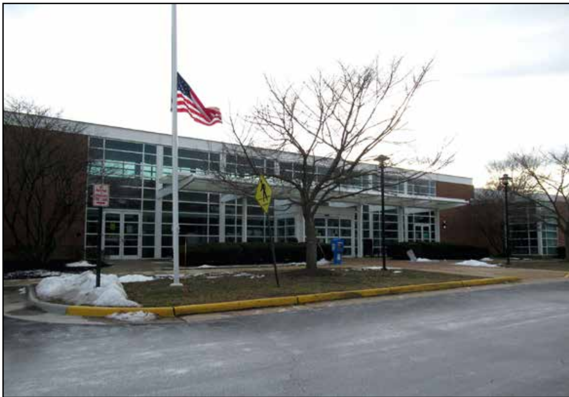
Figure 3.65. James Lee Community Center (029-6030), north entrance.
