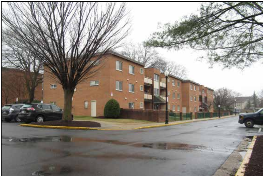
Figure 3.6. Bailey's Crossroads (029-6925), Oakview Apartments.
