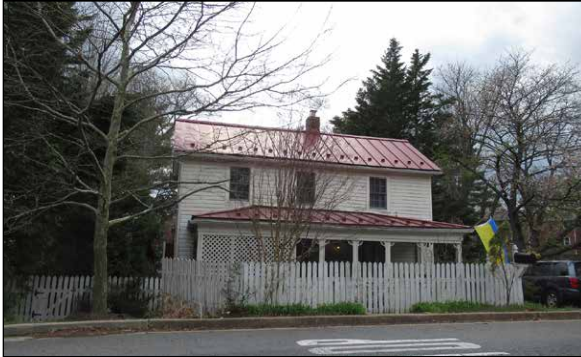
Figure 3.137. West End district (029-6942), Taylor House, 214 Nutley Street.
