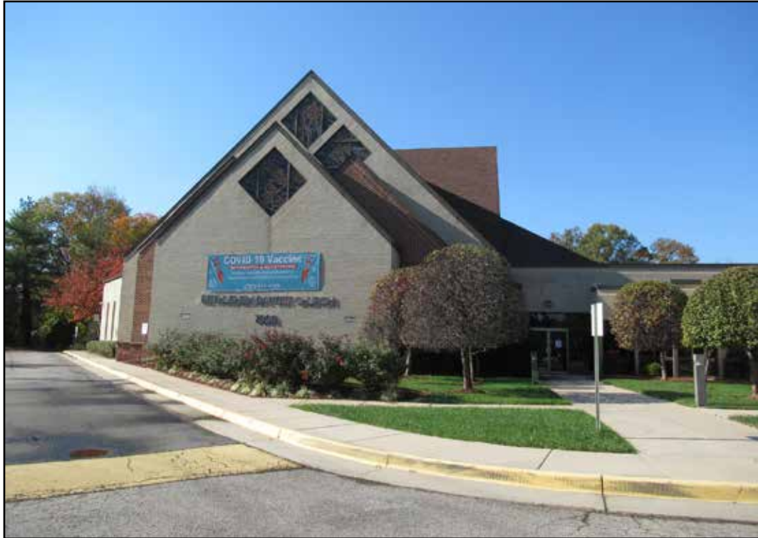
Figure 3.8. Bethlehem Baptist Church (029-6007), new church, facade.
