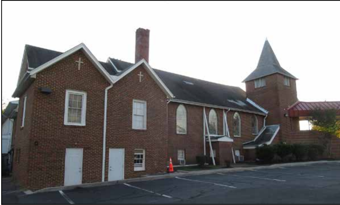
Figure 3.107. Second Baptist Church (029-6034), north elevation
