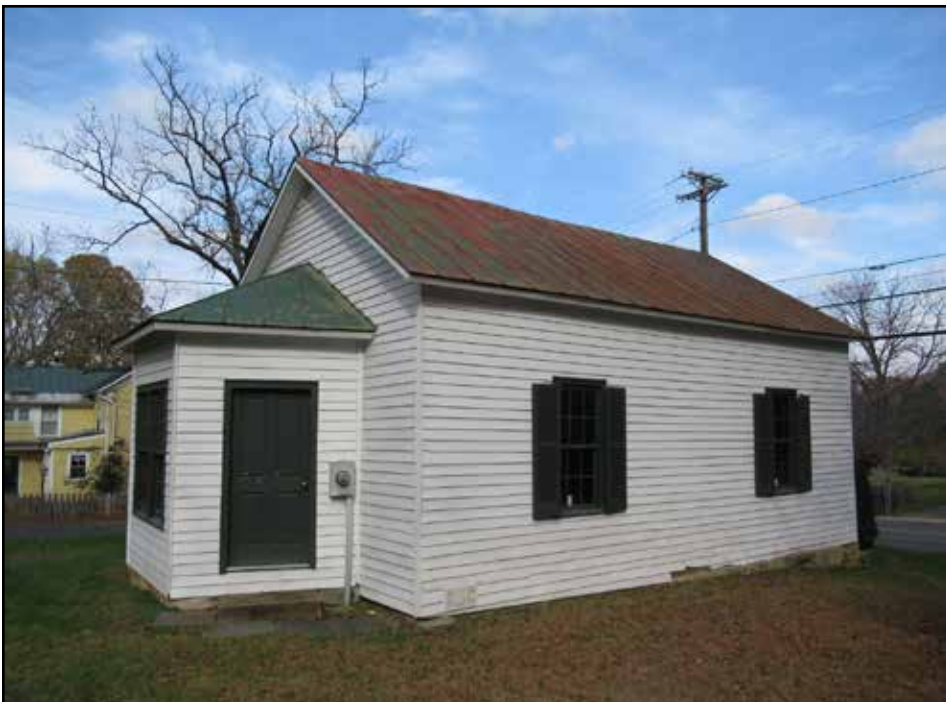
Figure 3.30. Clifton Primitive Baptist Church (194-0003-0024), south corner.
