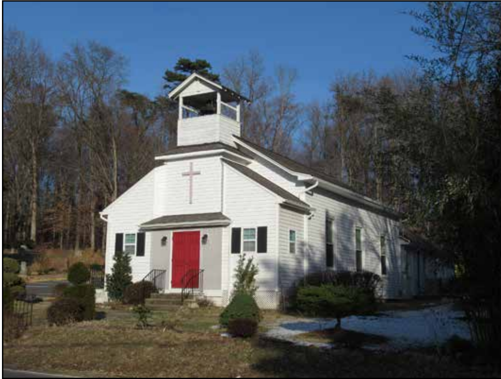
Figure 3.2. Accotink Methodist Church (029-5697), southwest corner.
