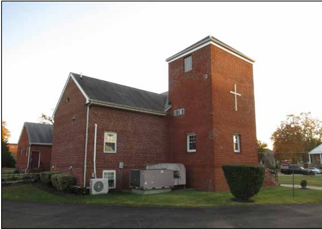
Figure 3.134. Warner Baptist Church (029-6889), north corner.
