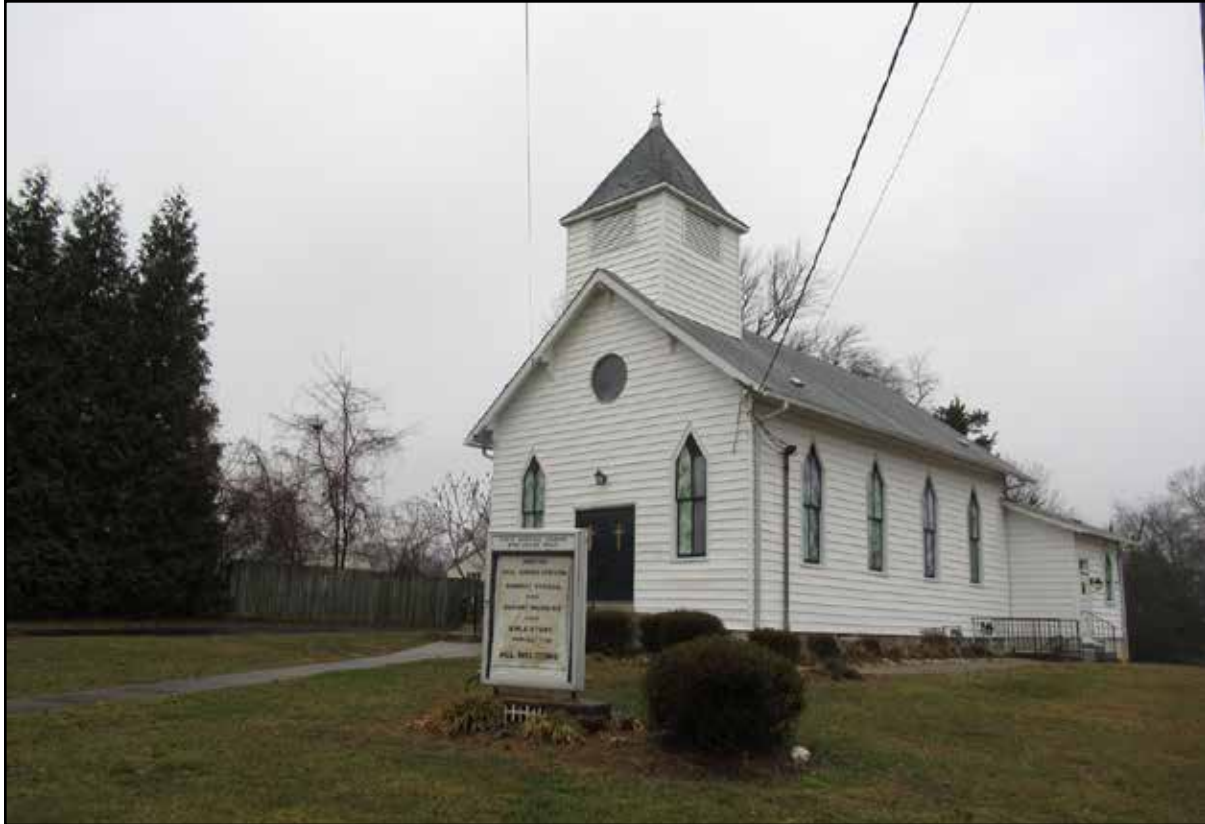
Figure 3.20. Chesterbrook Baptist Church (029-6029), east elevation.
