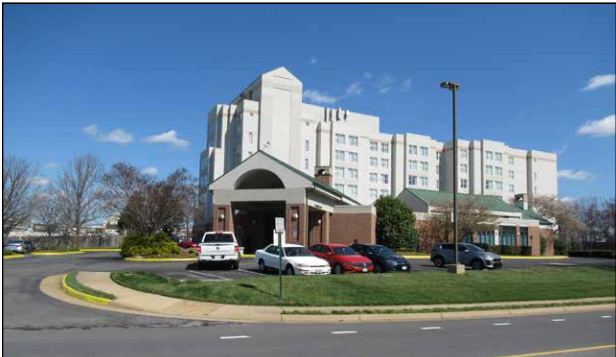
Figure 3.86. Merrifield area (029-6944), Porter Road, view to north.
