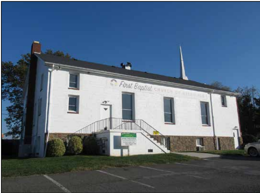
Figure 3.44. First Baptist Church of Merrifield (029-6888), west elevation.
