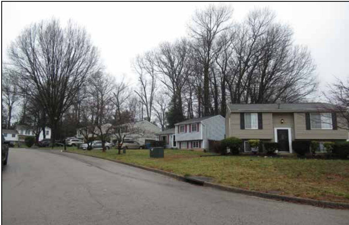
Figure 3.117. Sideburn area (029-6936), Laura Belle Lane, view to the south.
