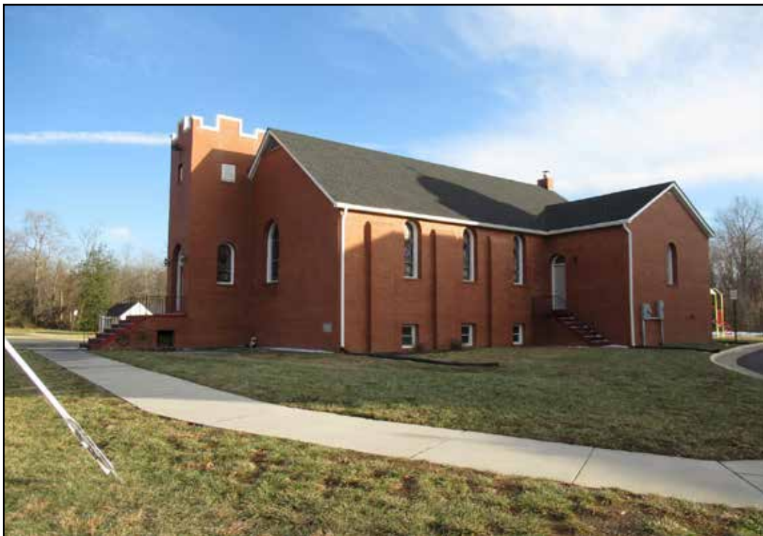
Figure 3.96. New Mount Zoar Baptist Church (029-6907), northwest corner.
