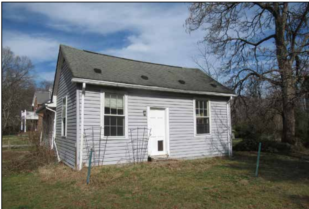
Figure 3.52. Gunston Hall area (029-6937), house on Harley Road.
