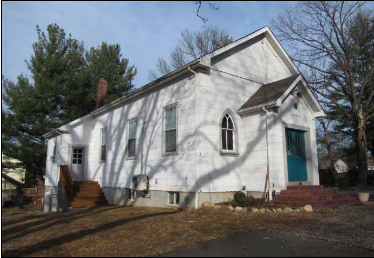
Figure 3.77. Little Zion Baptist Church (029-0376), southwest corner.
