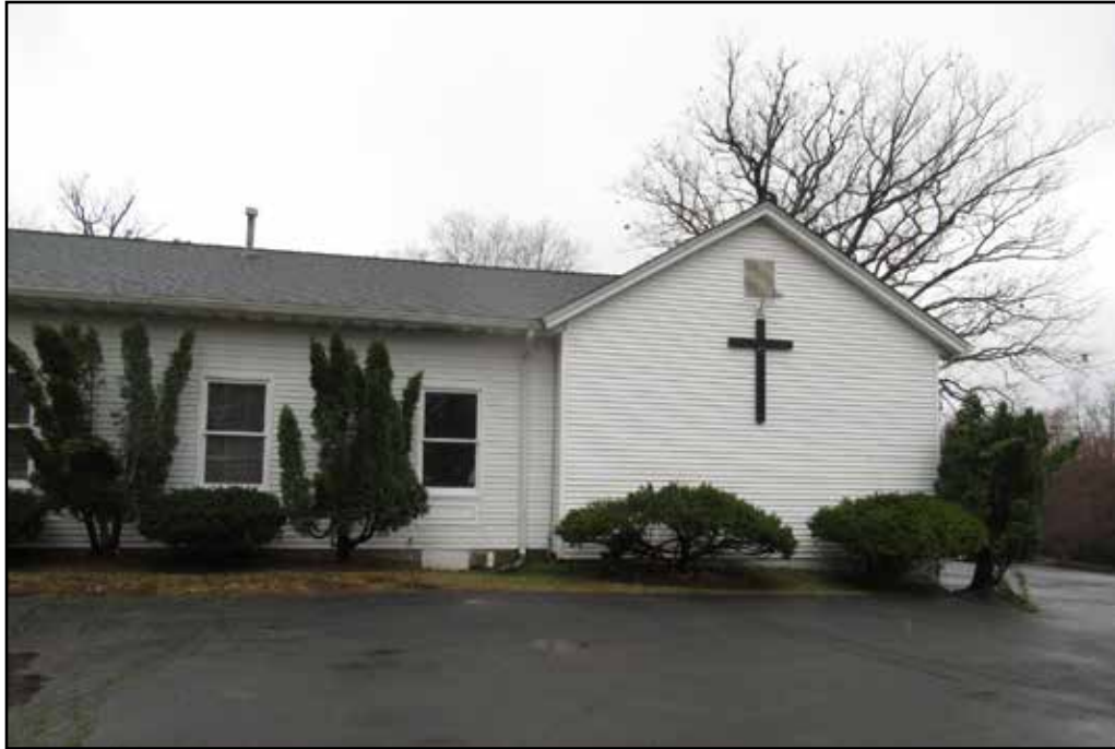
Figure 3.38. Cub Run Colored School/Centreville Assembly of God (029-6930), northeast elevation.
