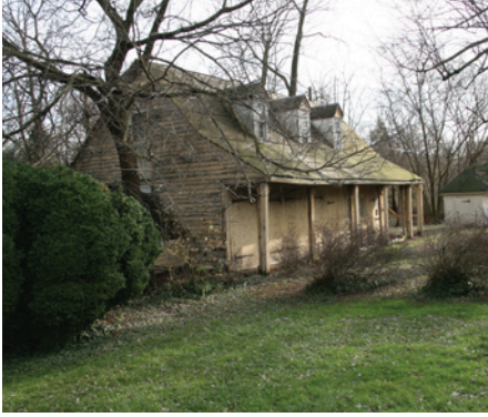
Historic outbuildings can provide additional examples for massing of new construction.
