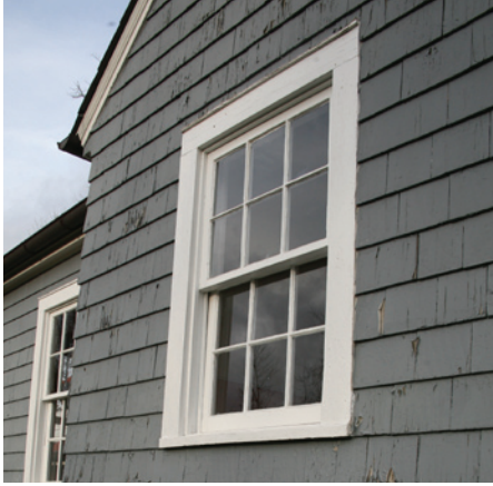
Six-over-six light windows are seen on the eighteenth-century Mount Gilead and on the Spindle Sears House.
