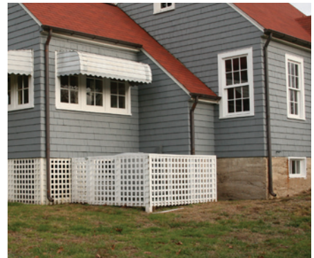
This lattice screen obscures the HVAC equipment for the house.
