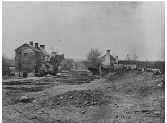
Taken from the opposite direction, this view shows a number of frame buildings which appear to be of a residential scale and form.
