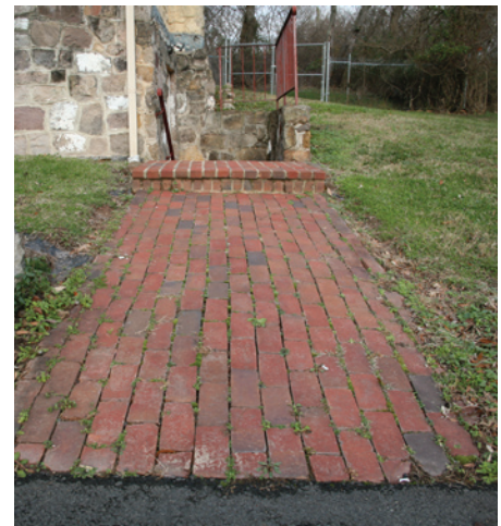
Brick and stone walkways found on residential sites within the district can be used as inspiration for new site elements.
