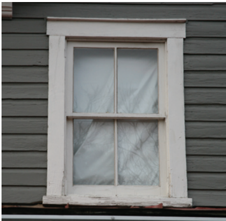
Two-over-two light windows were popular in the late-nineteenth and early-twentieth centuries as seen on the Enos Utterback House.
