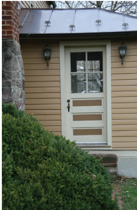
Examples of traditional materials such as the stone and brick chimney, clapboard siding, and standing-seam metal roof can be found on houses in the district including the Havener House as seen in this view at the rear of the house.
