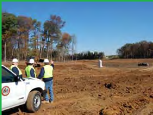
Soil filling on a development site to mitigate problem soil.
