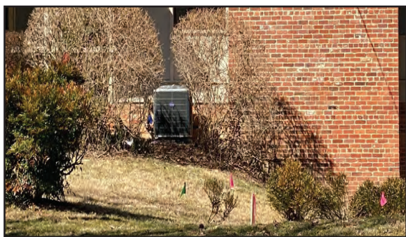
Placement of new systems in highly visible areas (not recommended).
