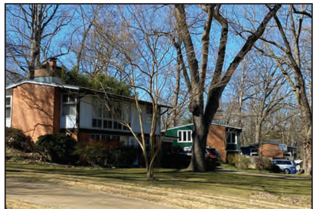
Low-slope side gable roof with wide exterior chimney and overhanging eaves (recommended).
