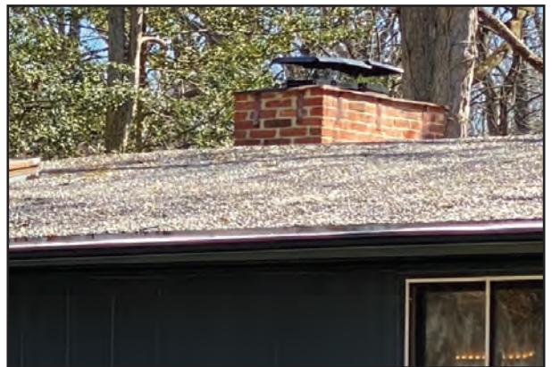
Low-slope gravel-clad side gable roof with low-profile gutters and internal brick chimney (recommended).
