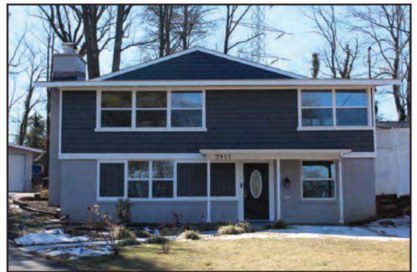
Original low-slope side gable roof modified to a more steeply pitched front gable roof (not recommended).
