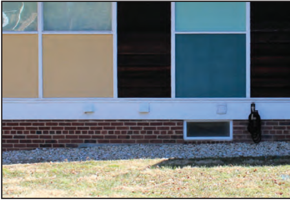
Low brick foundation, with plywood panels and horizontal wood siding above (recommended).
