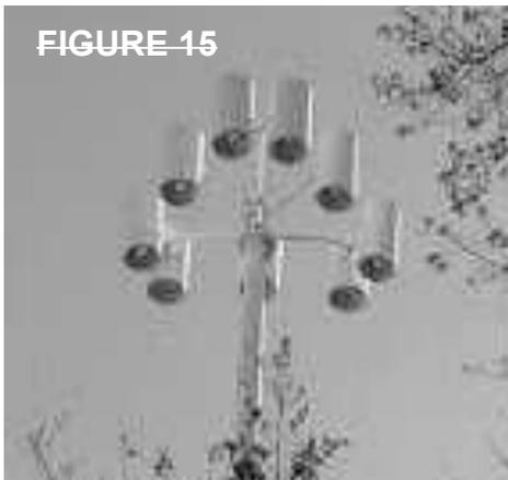
Antennas can be of a “candelabra” design and covered with a cylindrical shell to provide a unified, organized appearance.
