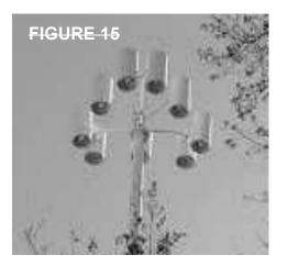
Antennas can be of a "candelabra" design and covered with a cylindrical shell to provide a unified, organized appearance.
