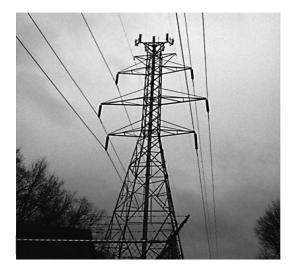
A "Fort Worth" structure integrates the telecommunication pole and antennas within an existing electrical transmission tower and helps to conceal the use. A 7 foot "radome cap" on the top of an electrical distribution pole conceals the telecommunication antennas.
