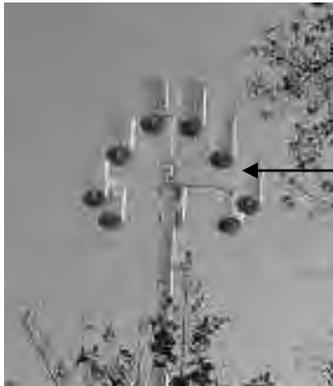
Antennas can be of a “candelabra” design and covered with a cylindrical shell to provide a unified, organized appearance.
