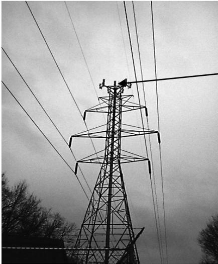
A “Fort Worth” structure integrates the telecommunication pole and antennas within an existing electrical transmission tower and helps to conceal the use.
