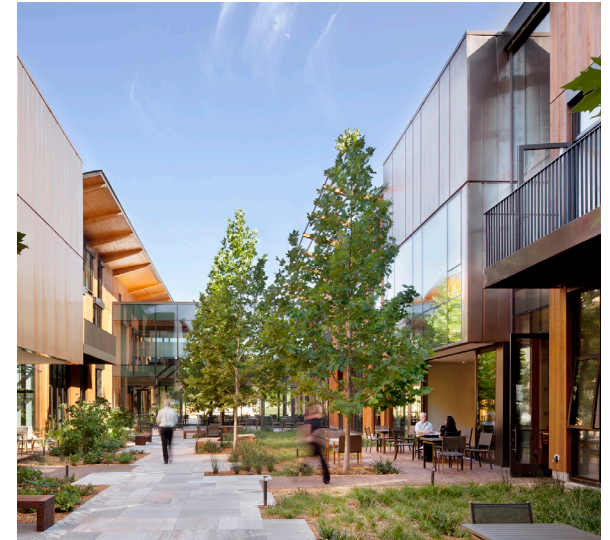
Linear Parks as Open Space Connections | David & Lucile Packard Foundation Building, Los Altos, CA | Image Credit: Jeremy Bittermann/EHDD
