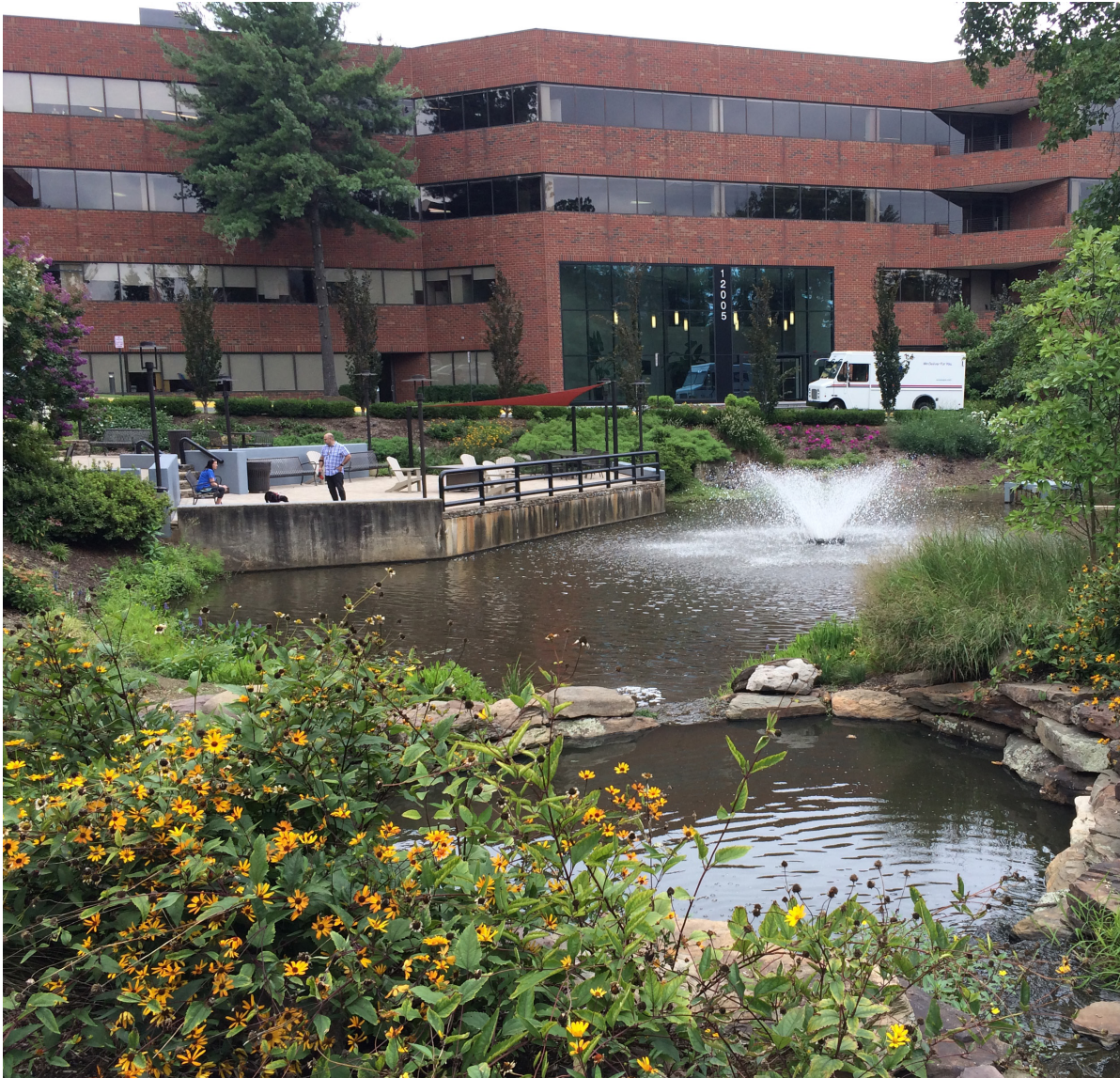
Office development around existing stormwater facility | Reston, VA | Image Credit: Fairfax County
