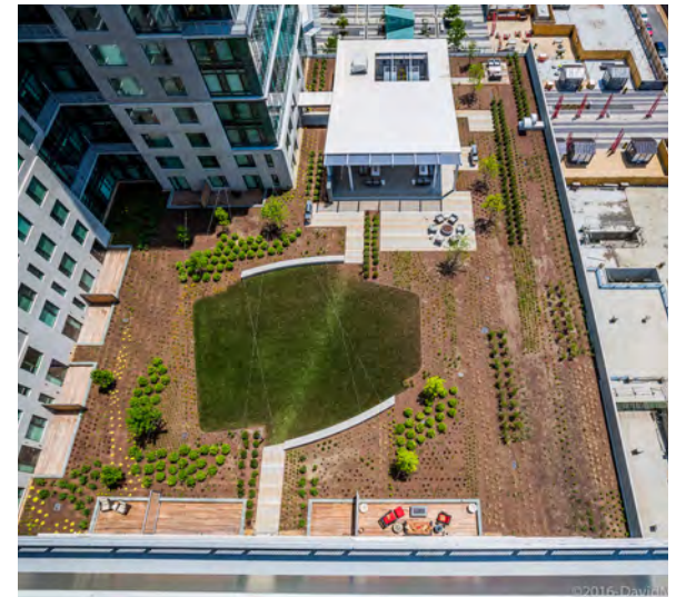
Green roof | Reston, VA | Image Credit: David Madison Photography
