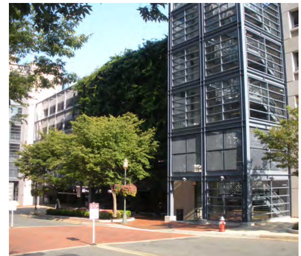
Parking garage screening option - Staircase access | Reston, VA | Image Credit: Fairfax County
