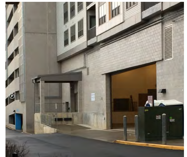
Utilities within building zone, service street | Fairfax, VA | Image Credit: Fairfax County
