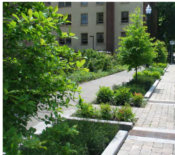
Vegetated stormwater management with tree/plant wells and swales | Portland, OR | Image Credit: City of Portland
