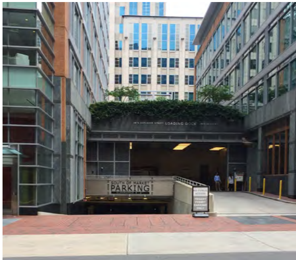
Below grade parking entrance co-located with loading | Reston, VA | Image Credit: Fairfax County
