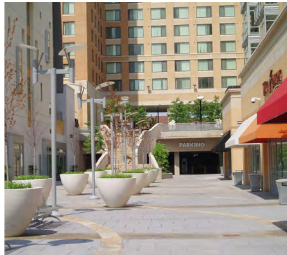
Co-located fire access with hardscape | Image Credit: Fairfax County
