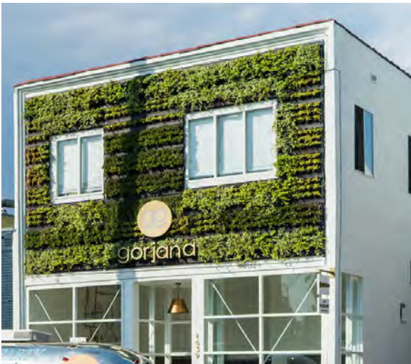
Vegetated wall on retail building | Venice, CA | Image Credit: Suite Plants
