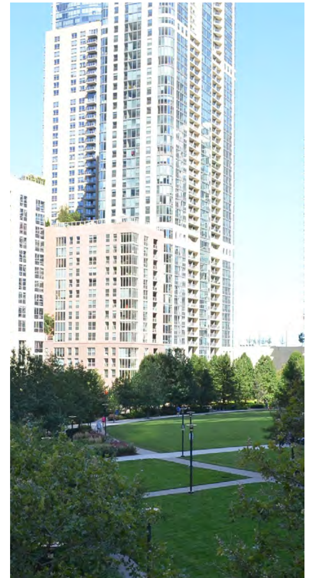
High-rise buildings oriented around a common green | Chicago, IL | Image Credit: Fairfax County
