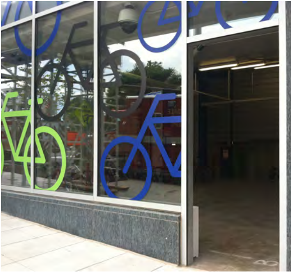
Indoor Bicycle Parking Facility | Reston, VA | Image Credit: Fairfax County
