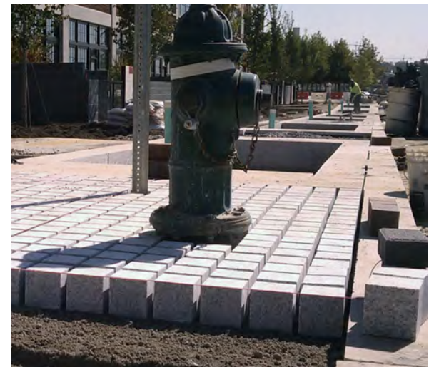
Permeable pavement installation in streetscape | Washington, DC | Image Credit: Fairfax County
