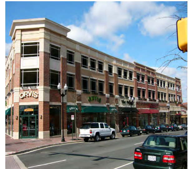
Parking garage with active retail ground floor and screening on the upper floors | Clarendon, VA | Image Credit: Fairfax County
