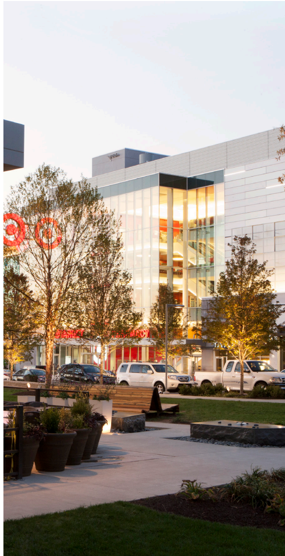
Building entry emphasized with projecting bay | Merrifield, VA | Image Credit: Edens
