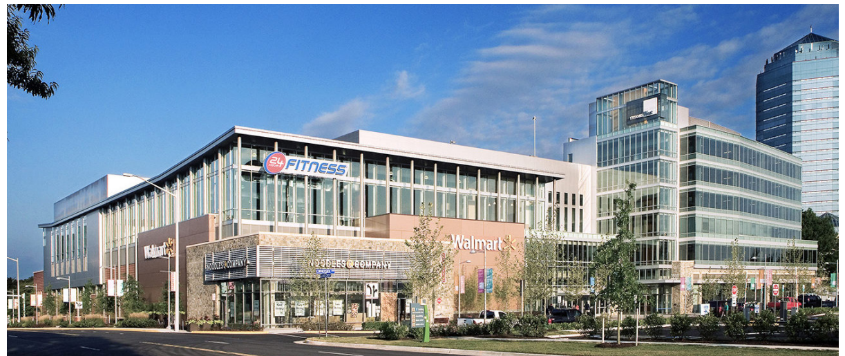
Articulate long walls and break buildings into a series of smaller masses | Tysons, VA | Image Credit: mv+a
