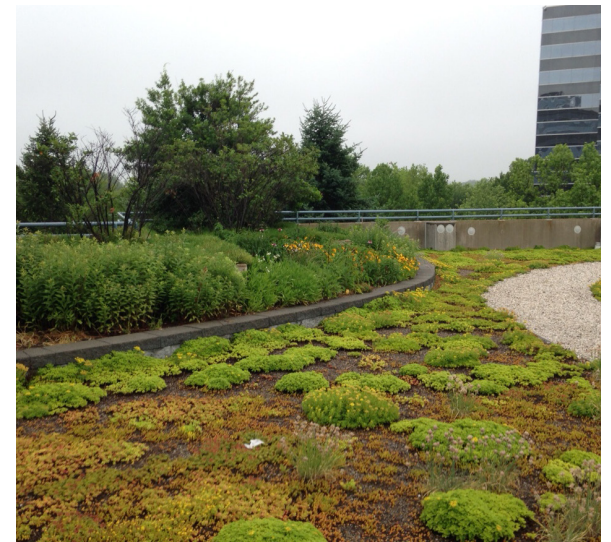
Green Roof Example | Fairfax, VA | Image Credit: Fairfax County
