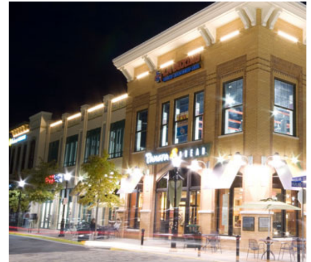
Upper floor fenestration | Reston, VA
