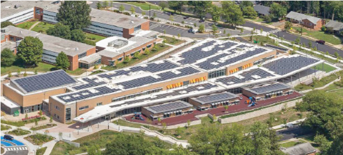
Large rooftop expanses are ideal for solar panels | Arlington, VA | Image Credit: Alan Karchmer Architectural Photographer
