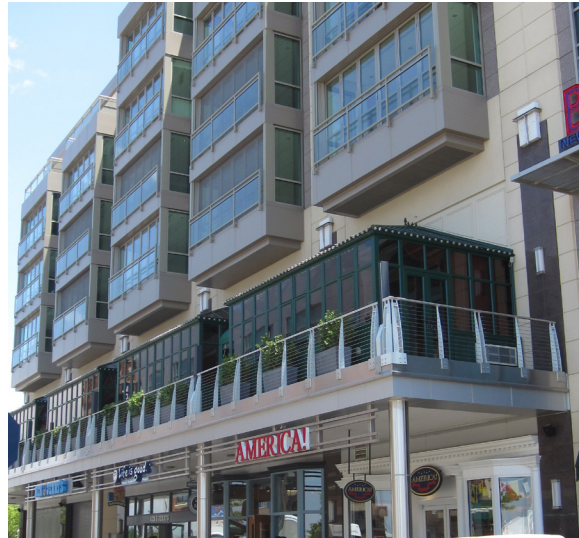
Building bump-outs | National Harbor, MD | Image Credit: Fairfax County
