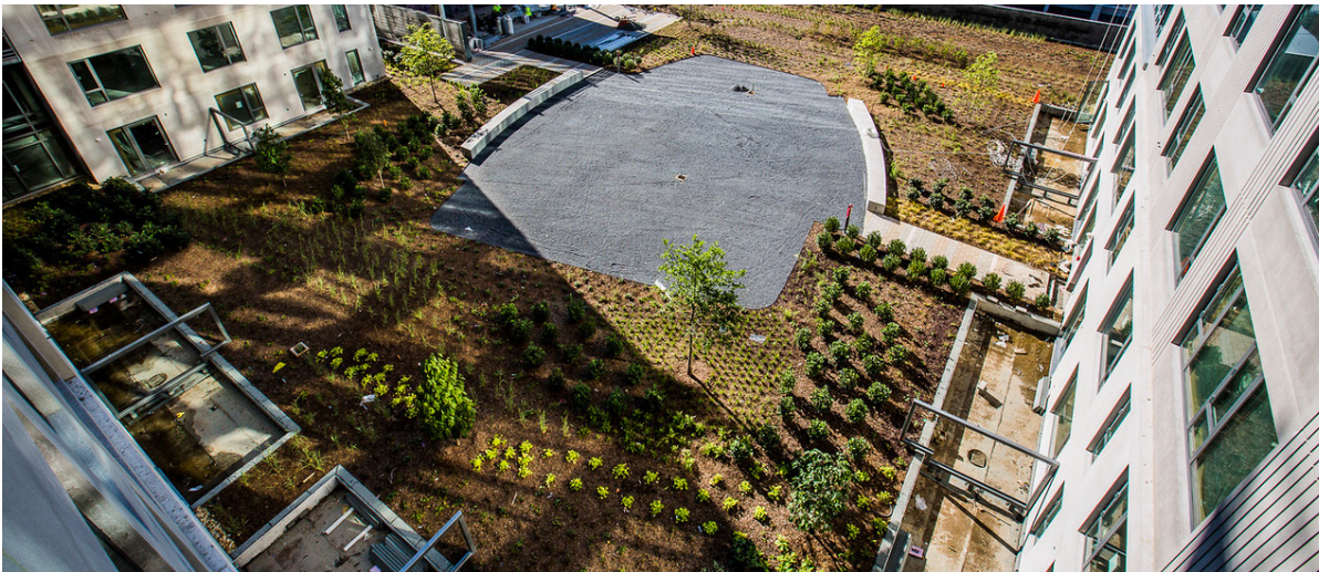
Green Roof Example | Reston, VA | Image Credit: David Madison Photography
