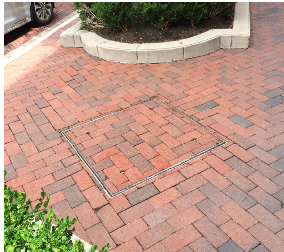
Utility access panel integrated into pavement design | Reston, VA | Image Credit: Fairfax County
