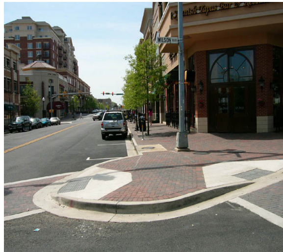
Bulb-out with dual pedestrian ramps | Arlington, VA | Image Credit: Fairfax County
