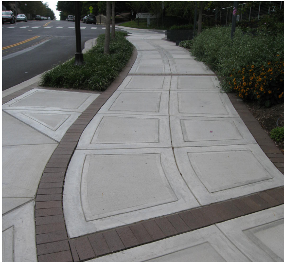
Scored concrete with pavers within the landscape amenity panel | Arlington, VA | Image Credit: Fairfax County
