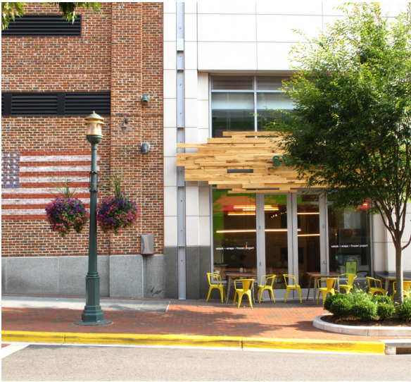
Streetscape example with active ground floor uses | Reston, VA
