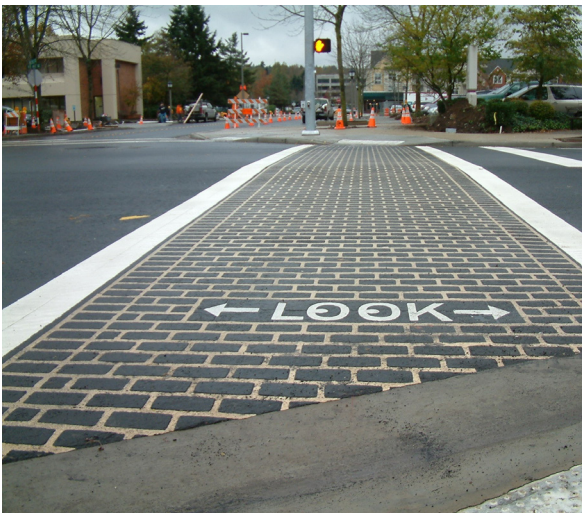
Graphics incorporated into crosswalk
