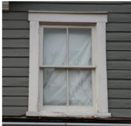
Two-over-two light windows were popular in the late-nineteenth and early-twentieth centuries as seen on the Enos Utterback House.
