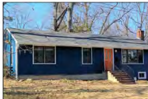
Foundation coated in concrete (not recommended)
