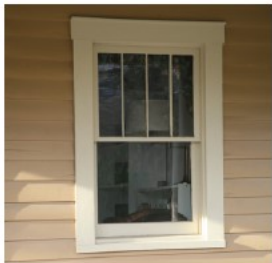
Multiple divisions in the upper sash over a single pane of glass below are seen on the Havener House.
