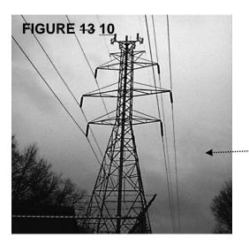
A "Fort Worth" structure integrates the telecommunication pole and antennas within an existing electrical transmission tower A 7 foot "radome cap" on the top of an electrical distribution pole conceals the telecommunication antennas.
