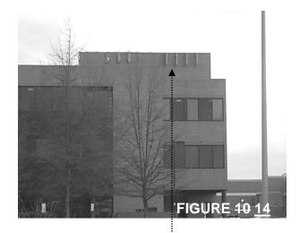
Place wireless telecommunication facilities to blend inconspicuously with existing structures. Place antennas "flush" against the building wall to blend with the building material.
