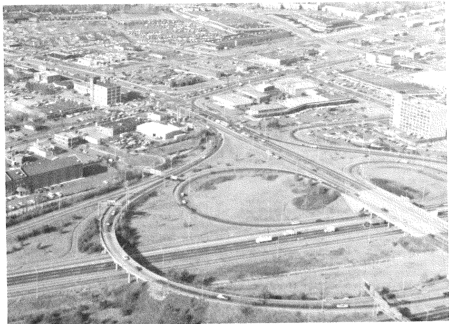
Old Keene Mill Road at I-95 looking northwest.
