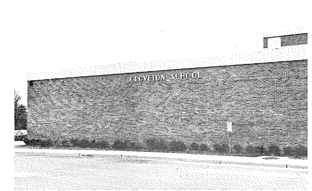
Groveton Elementary School, north of Huntley.
