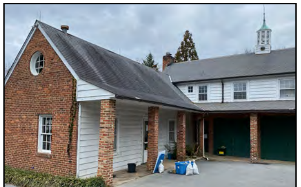
Gable roof with overhanging awning; note the cupola for ventilation and ornamentation.
