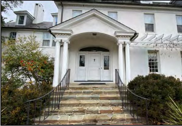
Primary entrance (paneled door) with sidelights, fanlight transom, and pedimented portico.
