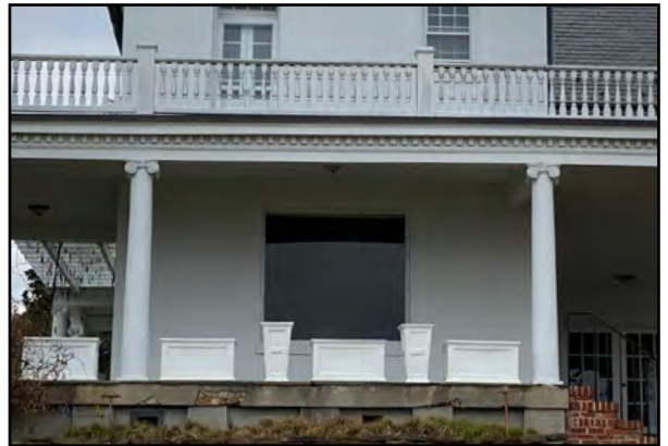
A large, single-light fixed window at the first-story of Wellington at River Farm that looks toward the Potomac. Fixed windows are atypical for Wellington at River Farm, and are not generally recommended.
