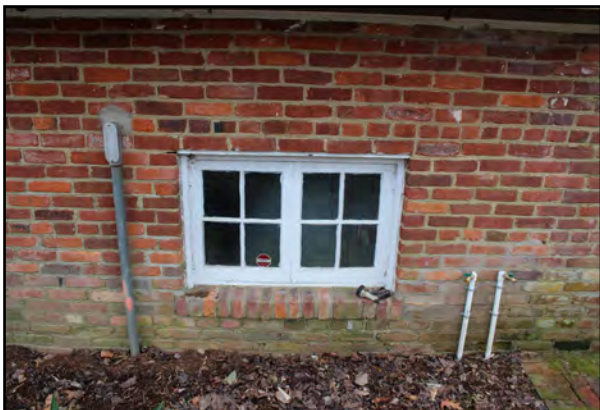
Brick cladding of the exterior continues to the foundation.
