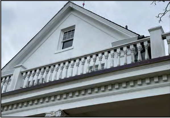
Detail of the dentilled cornice and balustrade of the porch; the gable end in the background has a full entablature.
