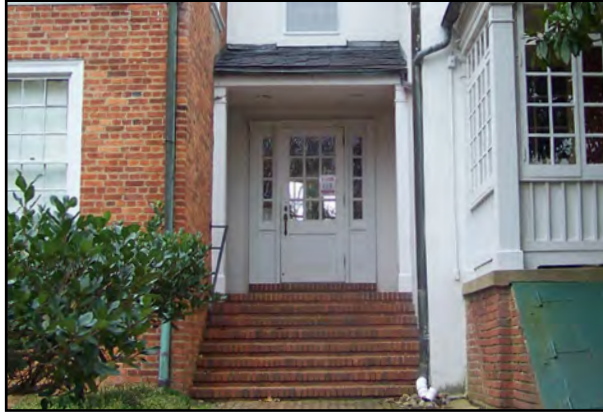
Secondary entrance beneath an entry stoop features a multi-light paneled wood door with sidelights.
