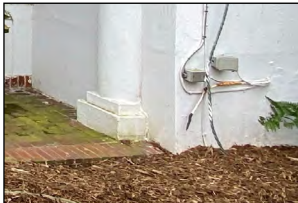
Parged masonry exterior used to cover and protect the exterior wall and foundation.
