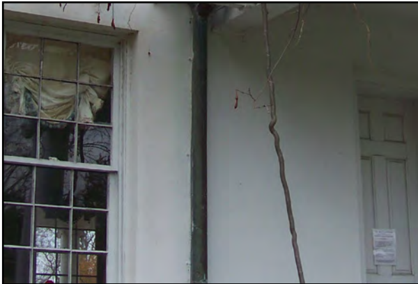
Brick masonry with applied stucco coating exterior of the main house at Wellington at River Farm
