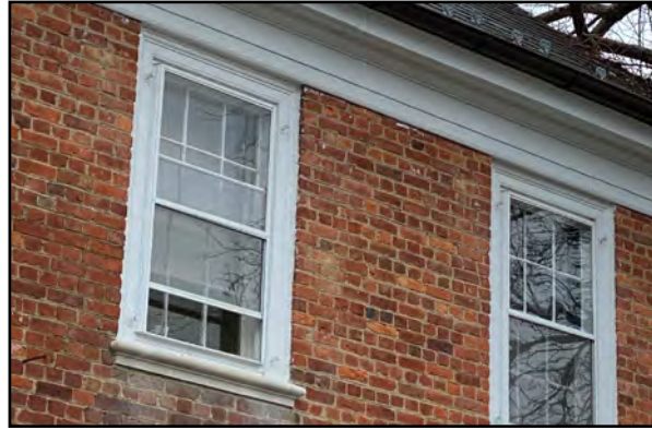
Double-hung windows, the most common type at Wellington at River Farm and typical of the Colonial revival style
