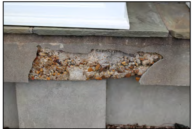
Deteriorated stucco coating on large aggregate concrete masonry
