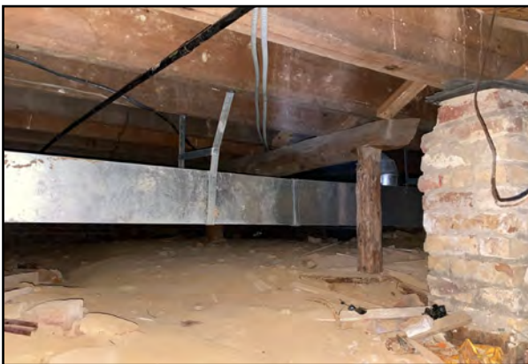
Modern ductwork added beneath the first floor framing
