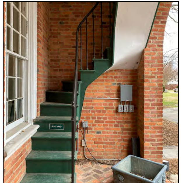
Half turn stair with iron rail located at the end of the arcade in the north wing.
