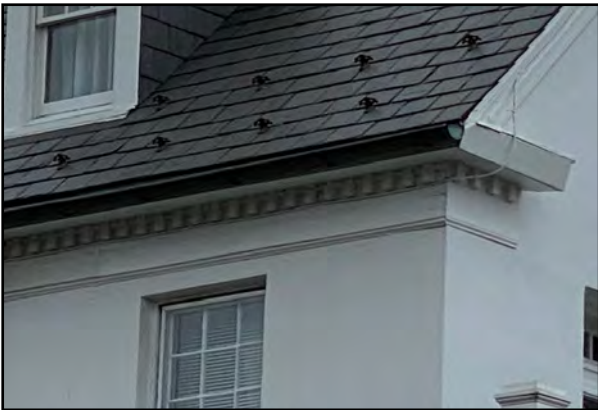
Dentilled cornice terminating at right with an eave return at right.
