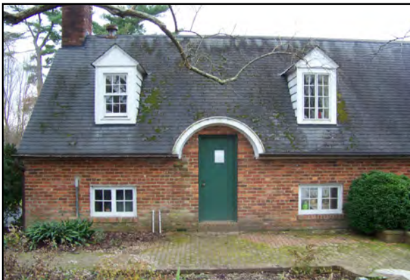
Side gable with dormers and arched hood over doorway.
