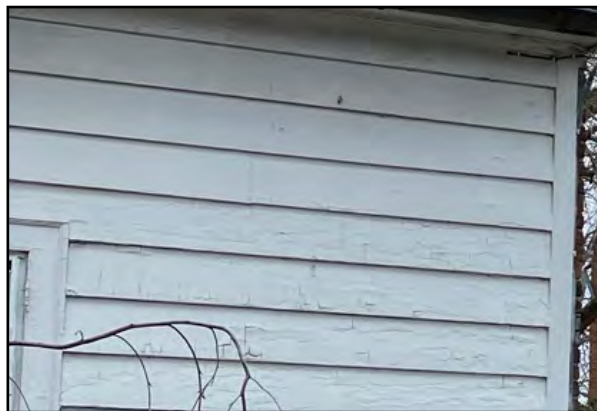
Wood weatherboard siding is used in combination with brick cladding on the stable or carriage house
