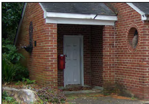
Entrance within a recessed entry stoop incorporated beneath the primary roof
