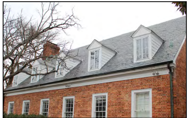
Standard gable roof with exterior end chimney and gable dormers
