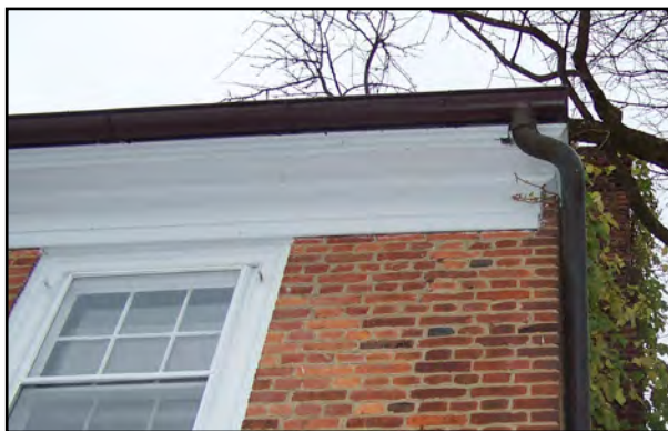
Detail showing soffit and wood fascia beneath the roof eaves.
