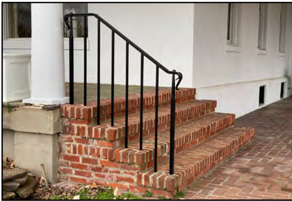
Cast iron railing on brick stairs leading down from the porch to the colonnade
