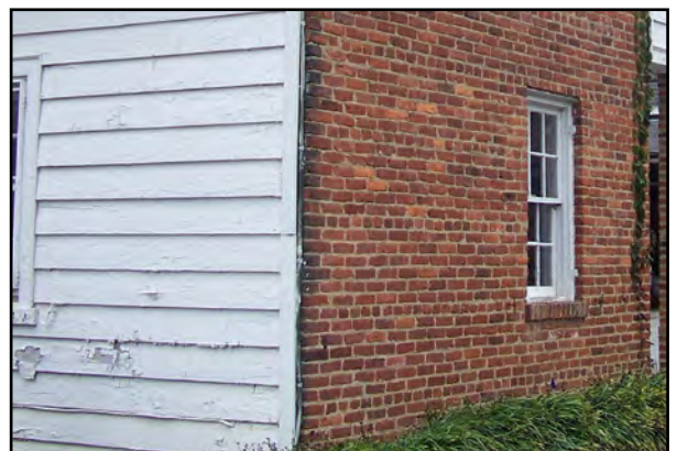
Wood weatherboard and brick, both common siding types, are sometimes paired on the same building
