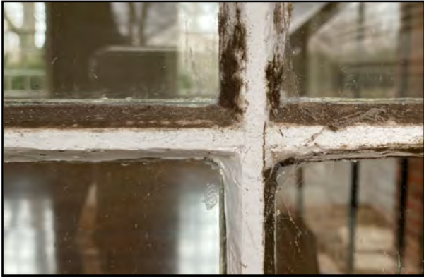
Detail of muntins holding window panes in place.
