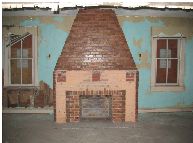
View of fireplace constructed with prison era brick. (101-1)
