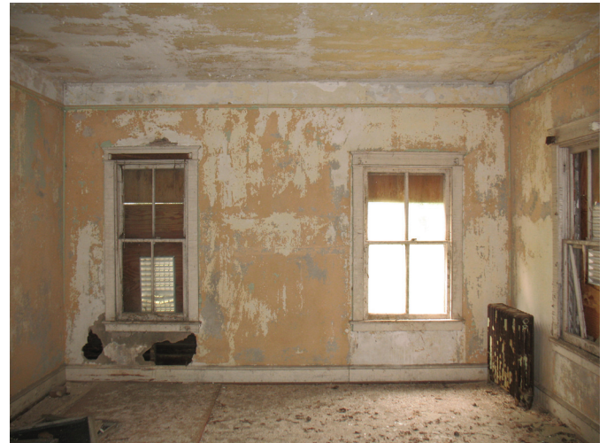
View of windows on north side of rear addition. Note indications in base and plaster of right window being converted from door to window. (102-2)
