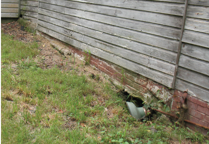
View of hole in foundation on south side of building. (X16)
