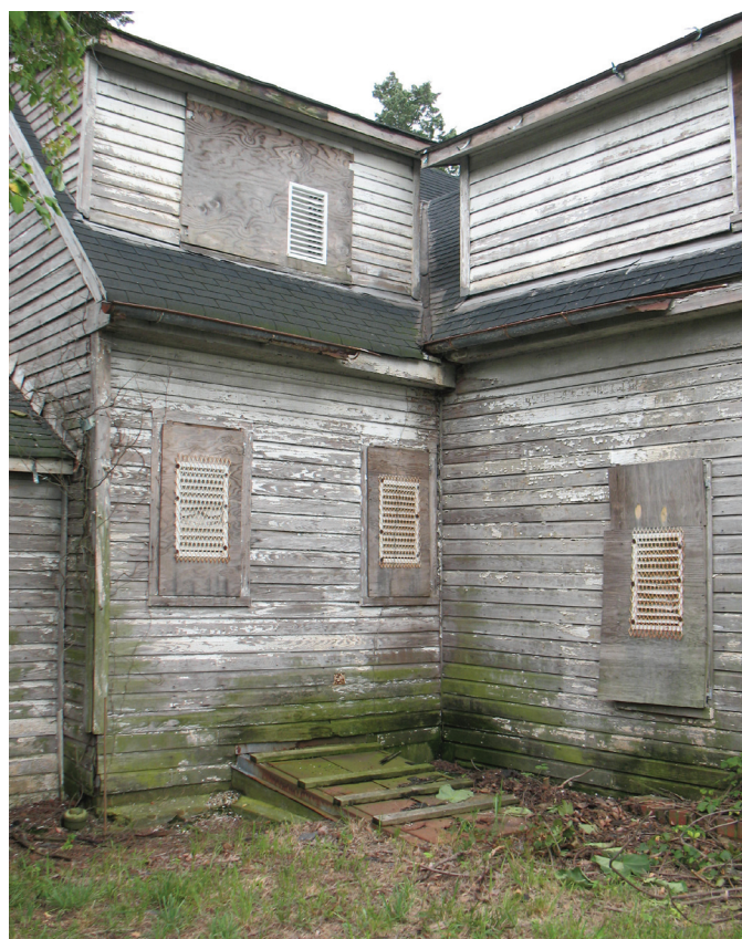
Close-up detail of building from northeast side that shows beveled siding on the dormers and German siding on the wall of the original house and addition. (X9)
