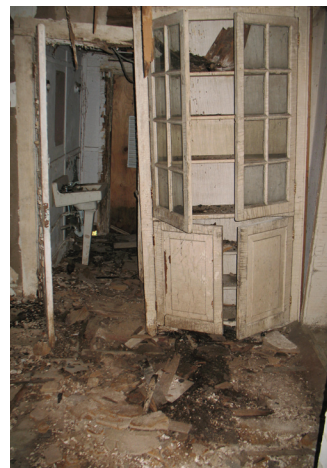
View of Room 106 facing bathroom to south. Note water damage to floor and built-in cabinet. (106-1)
