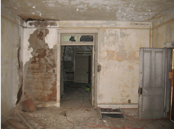
View of rear door to original section of house. Note later wire mesh over German siding at area of water damage to left of door. (102-1)
