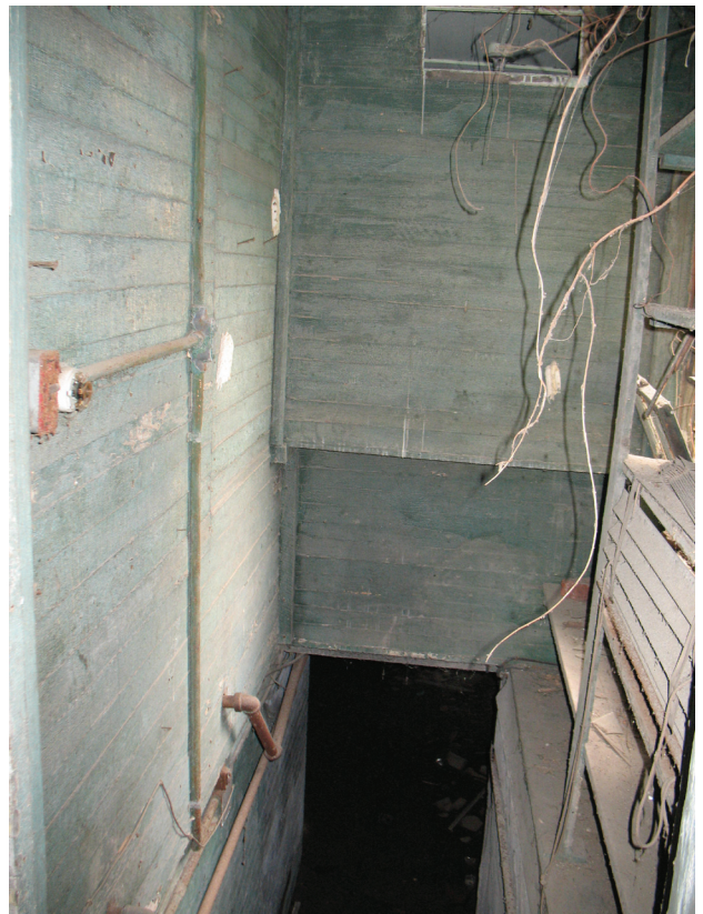
View of board wall finish in stair. (108-1)
