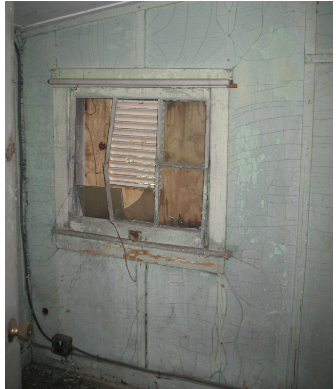
View of casement window and hardboard wall finish. (110-1)
