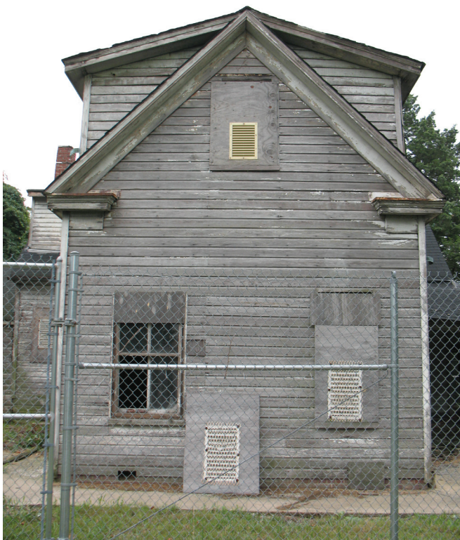
Close-up view of rear addition from north side. Note shed dormers and classical cornice with returns. (X7)
