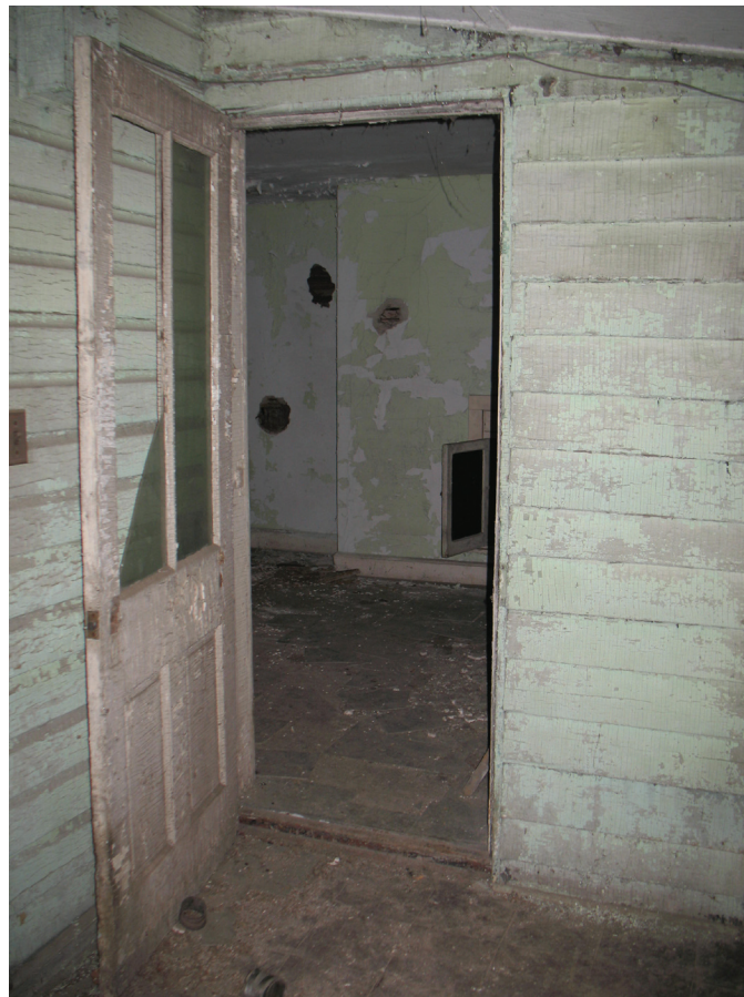
View into room 106 from room 109. Note German and clapboard siding on the south and west walls, respectively. (109-1)
