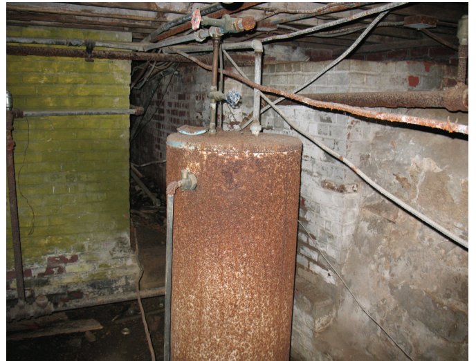
Basement view facing southeast. Note transition from stone to prison-era bricks in foundation wall. (B01-10)
