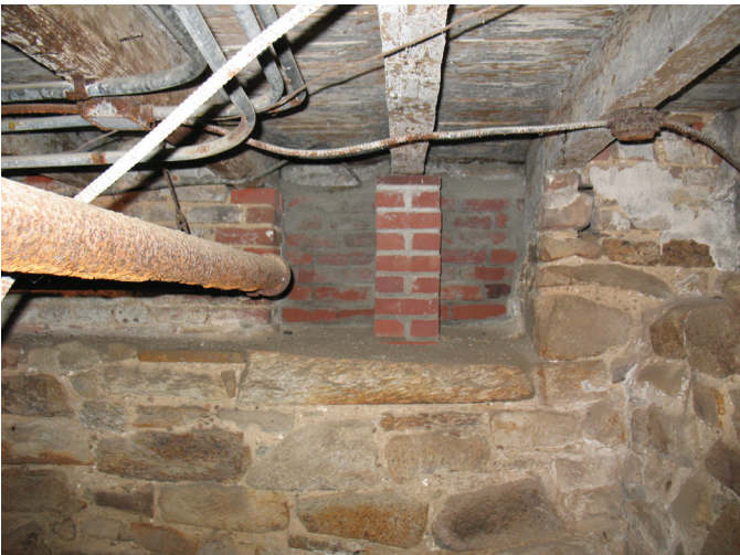
Basement view of brick pier added at window opening on south side of foundation. (B01-5)
