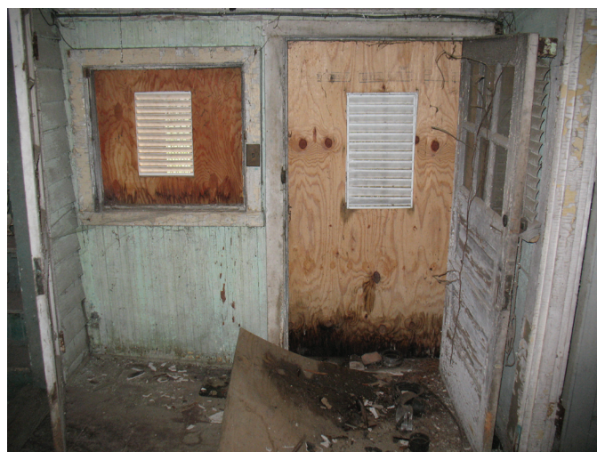
View of exterior door and tongue-and-groove wood wall finish. (109-2)
