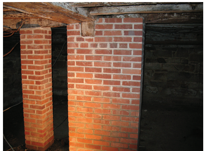
View of supplemental brick piers added in basement. (B01-3)
