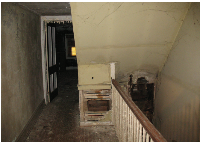
View toward room 202 at rear of house. Note location of likely original chair rail and base on section of wall missing plaster. (203-3)
