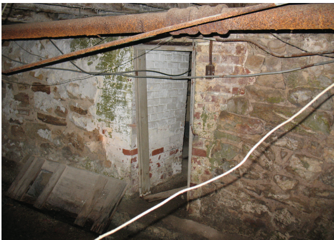
Basement view of door to small room added to north side. Note prison-era bricks used to create door opening in stone foundation. (B01-2)
