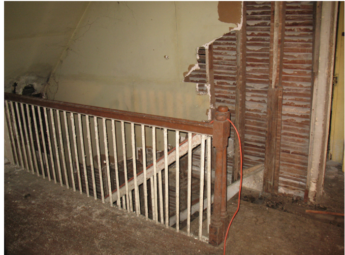
View of likely original railing in second floor hall. Note double newel post. (203-1)
