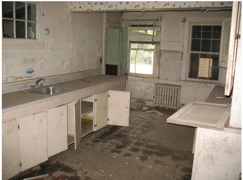
View toward east end of kitchen showing finishes dating from mid-twentieth century. Note casement window on interior wall above countertop. (112-2)
