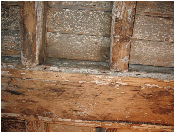
Basement detail of original sawn floor joists, hand-hewn summer beam and plank floor above. (B01-1)
