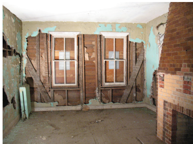
View of west wall with braced timber frame exposed. (101-2)
