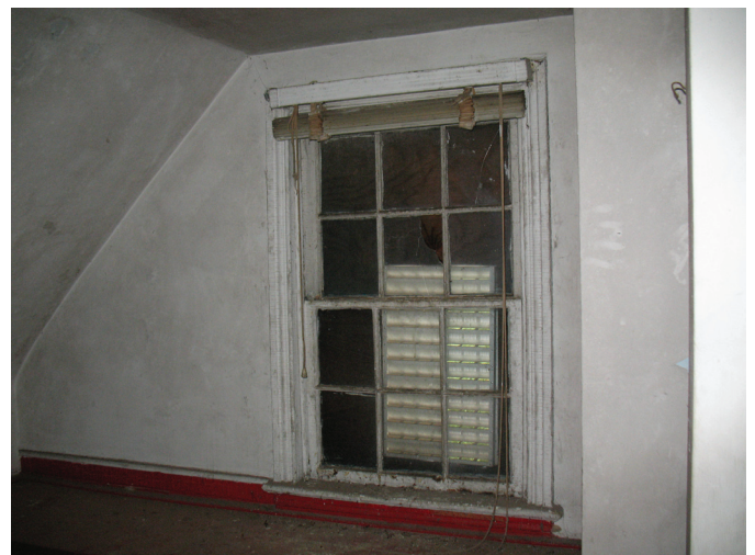
View of window in gable end of house. Note the six-over-six light pattern and molded trim. (201-3)
