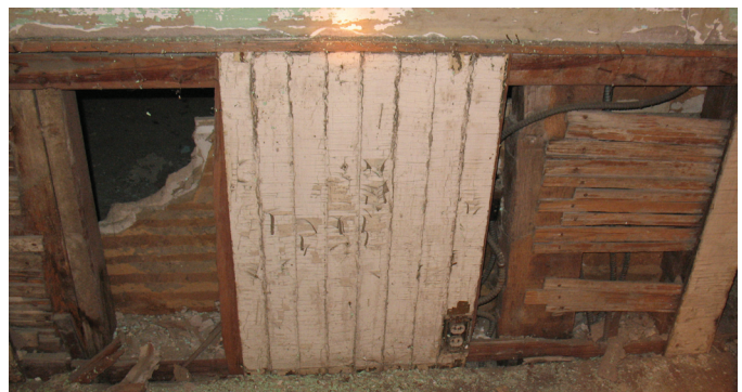
Detail view of remaining split wood lathe and original base and chair rail in original hall. (103-3)
