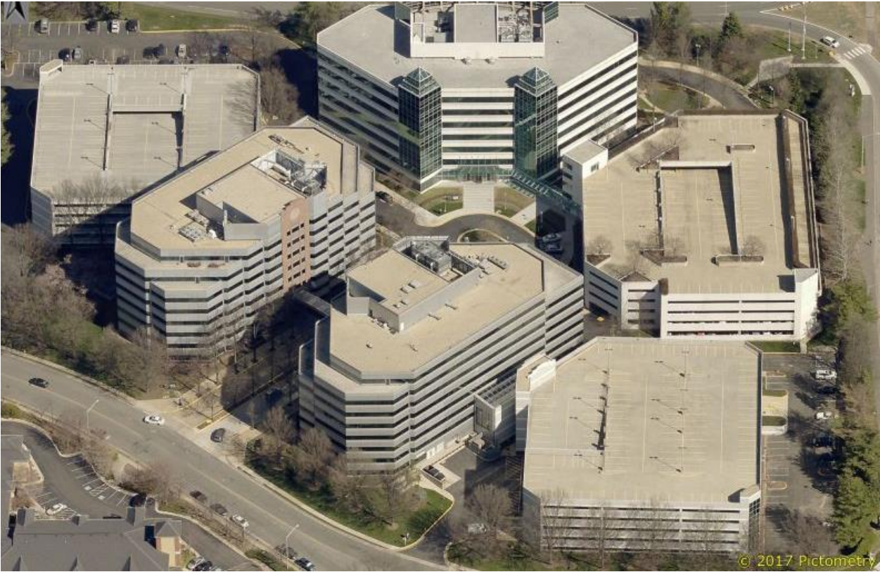
Figure 2103.5: C-3 District Aerial Example
