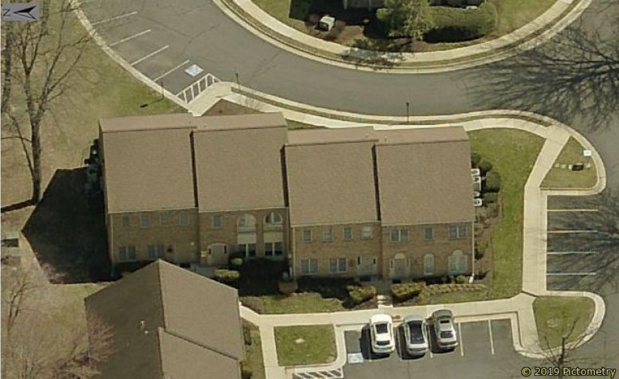
Figure 2103.1: C-1 District Aerial Example
