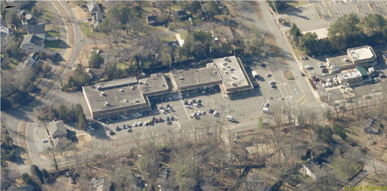
Figure 2103.9: C-5 District Aerial Example
