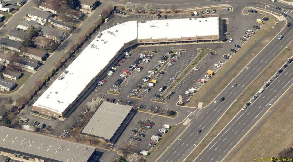
Figure 2103.15: C-8 District Aerial Example
