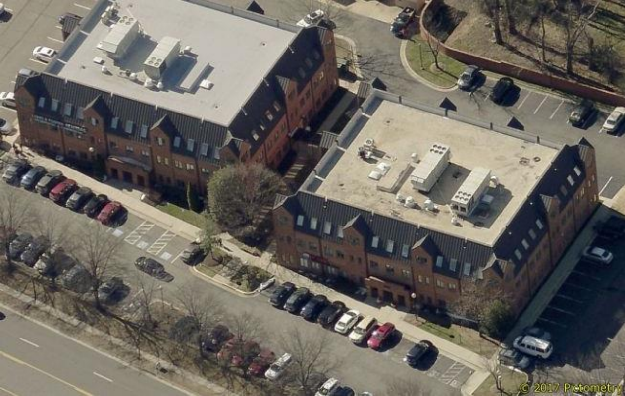
Figure 2103.3: C-2 District Aerial Example
