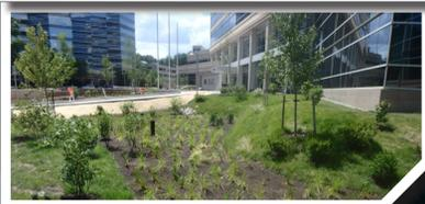
These depressed, landscaped gardens capture and filter stormwater runoff. During storms, runoff temporarily ponds then rapidly filters through a bed of sand, soil, and organic filtering media. Native plants like rushes and sedges help take up and treat stormwater, provide wildlife benefits, and create appealing landscaping.
