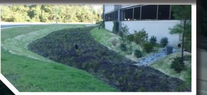
Vegetated swales provide the same services as bioretention cells, but they are shallower, configured as linear channels, and can be planted with sod or native plants. These swales create a 1,100-foot-long treatment path that terminates at an engineered outfall.
