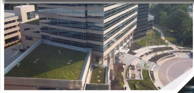
Five vegetated roofs use special drainage systems to slow down, evaporate, and filter rainwater before it enters the drain. Green roofs also moderate internal temperatures.
