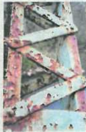
Bridge corrosion photo by Jim Palmer.
