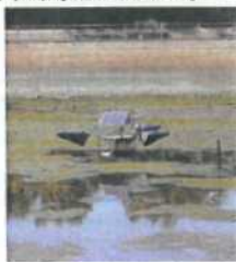
Solar mixer at Noman M. Cole, Jr. Pollution Control Plant
