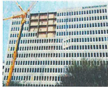
Removal of Precast Façade - 7900 Westpark Drive
