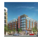
Founders Row Falls Church, VA Type IIIA wood construction over Type I concrete podium and some Type V
