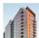
Gallery Bethesda I Bethesda, MD Certified LEED-NC Gold
