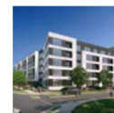
Riverside Alexandria, VA Type IIIA wood construction over Type I concrete podium
