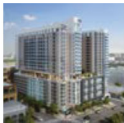
Modera Buckhead Atlanta, GA 21-story apartment building with 398 units and 20,000-sf retail
