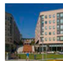
Terrapin Row College Park, MD Type IIIA wood construction over Type I concrete podium
