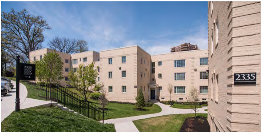
Woodbury Park Apartments 349,300 gsf / $31M
