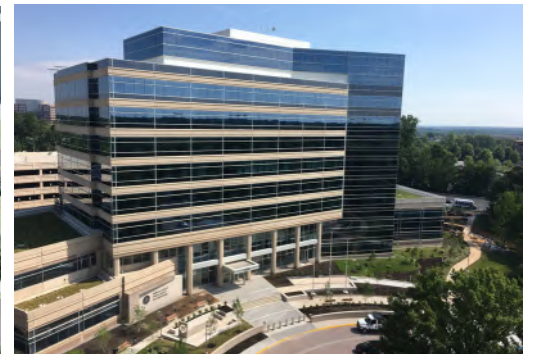
Fairfax County Public Safety Center Fairfax County, VA
