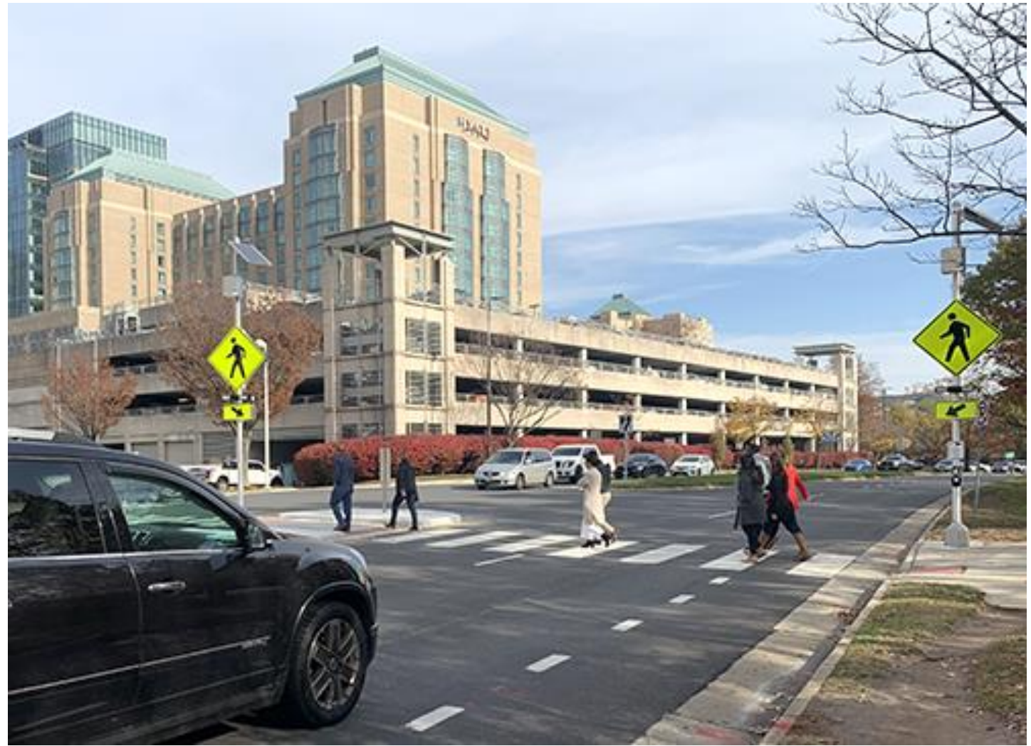
RRFB at Bluemont Way and Discovery Street in Reston, Virginia
