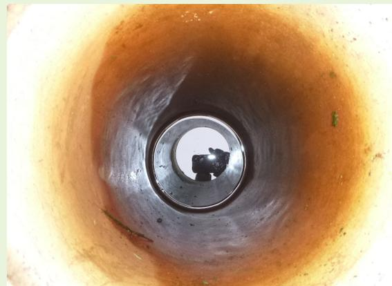
Photo 4 - Standing water observed inside observation well for more than 48 hours.
