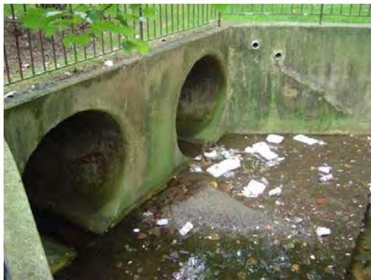
Outlets filled with trash and debris
