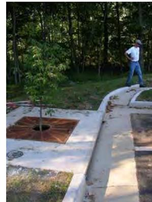
Newly constructed parking lot with existing tree box filter, underdrain, and infiltration
