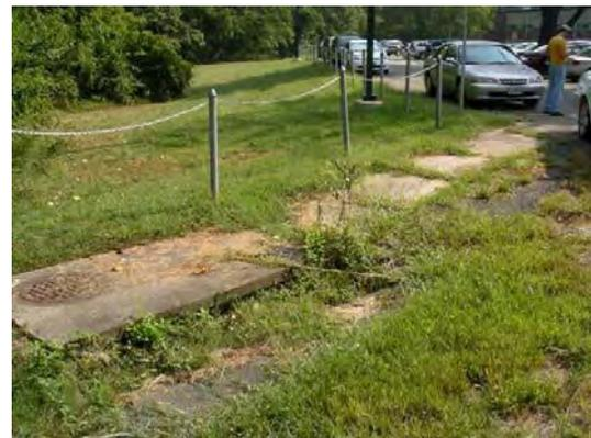
Potential bioretention area at stormwater inlet
